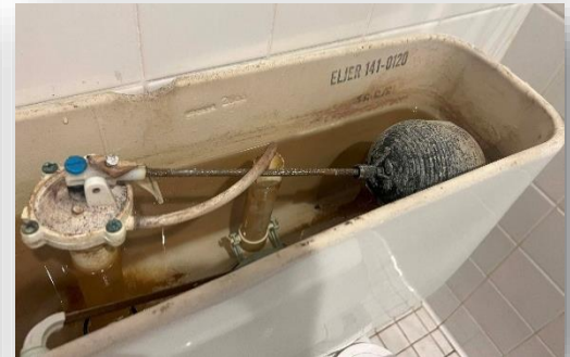
Checking the refill and overflow tubes in toilet tanks for proper settings.
