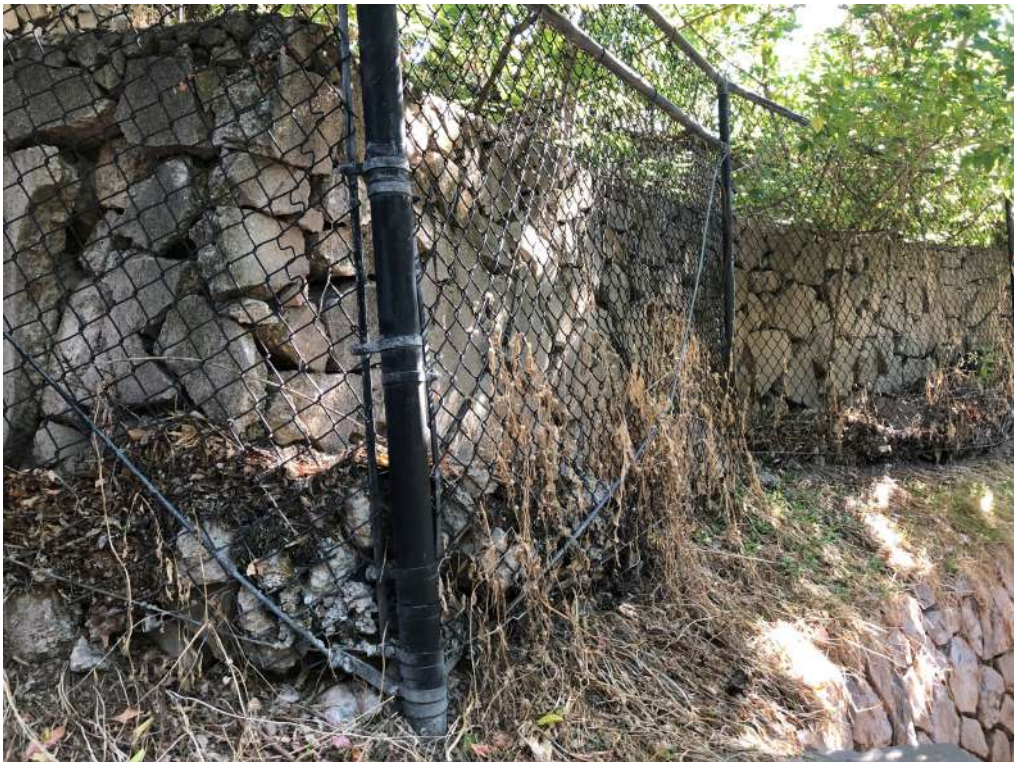
Photograph 4 - Retained slope constructed above the top of the rock wall.
