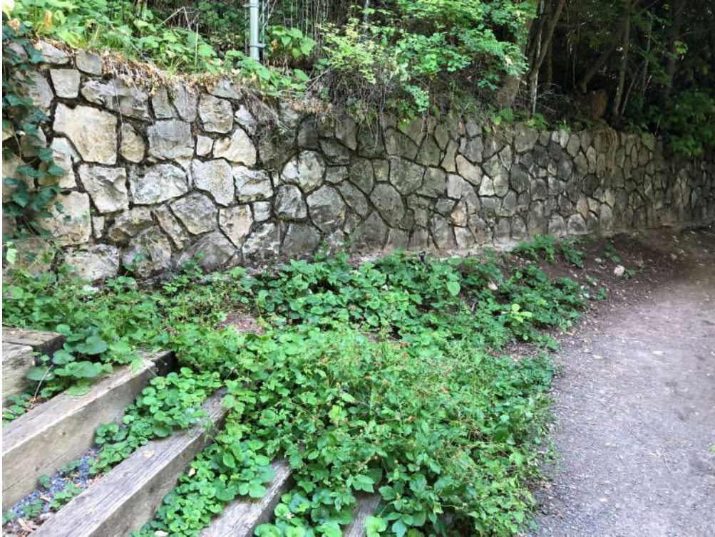
Photograph 5 - Ground below the rock wall has been lowered.
