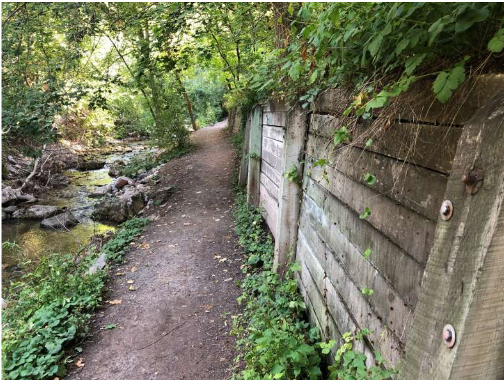
Photograph 8 - Timber wall section appears to have rotated away from slope.
