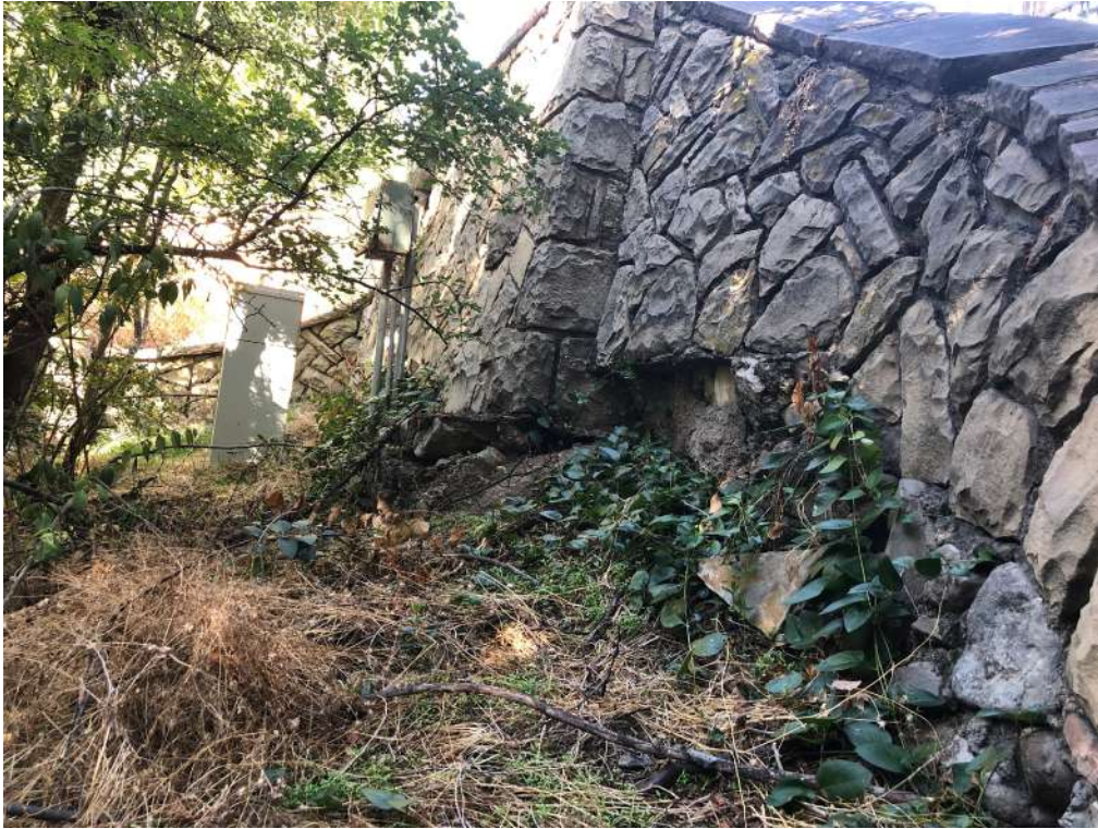
Photograph 1 - Undercut wall near the north park entrance at 900 South.
