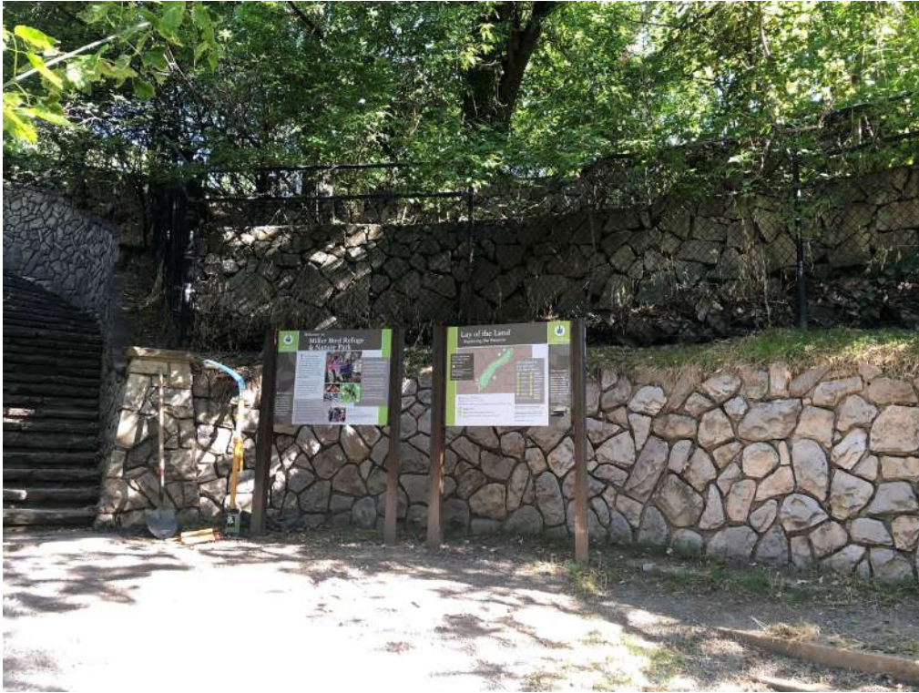
Photograph 3 - Retained slope constructed above the top of the rock wall.
