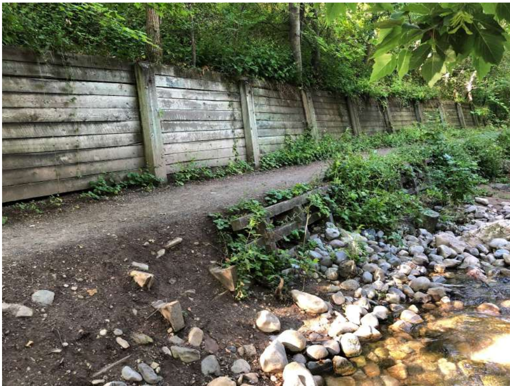
Photograph 10 - Crib wall on east side in poor condition. Timber wall above appears bulging or rotating.
