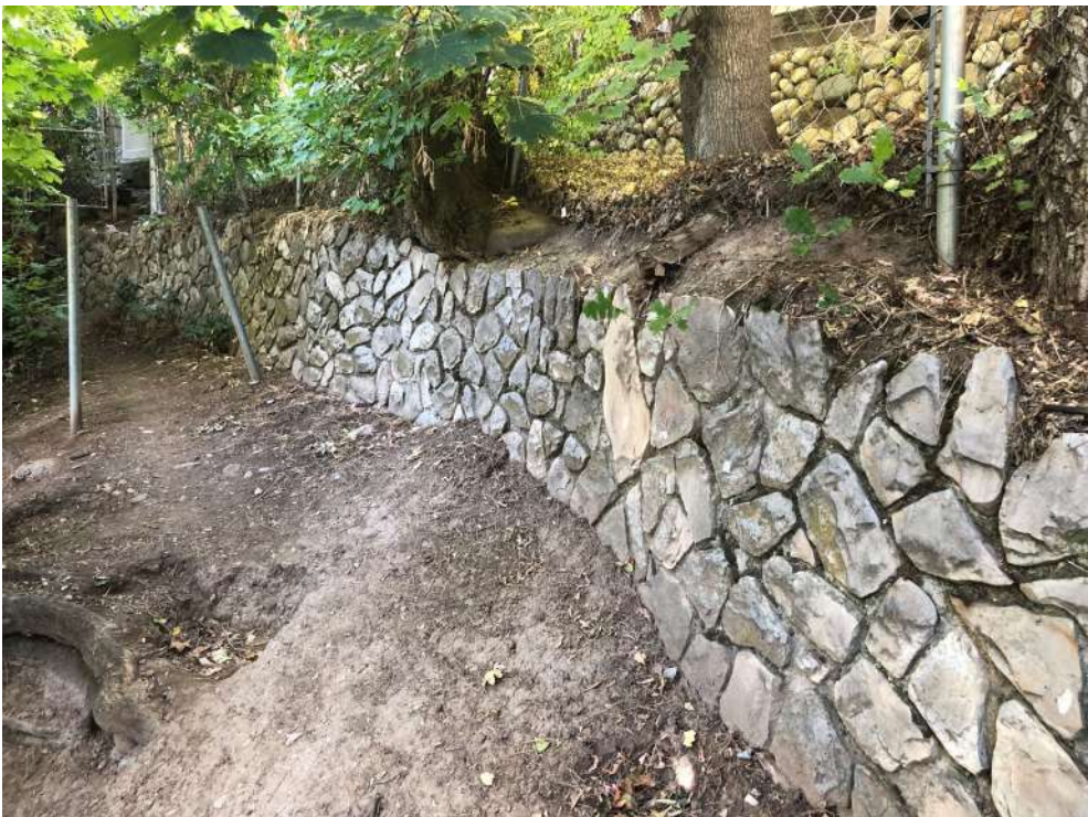
Photograph 12 - Rock wall above the area of erosion. Note trees and other loads near the top of the wall.
