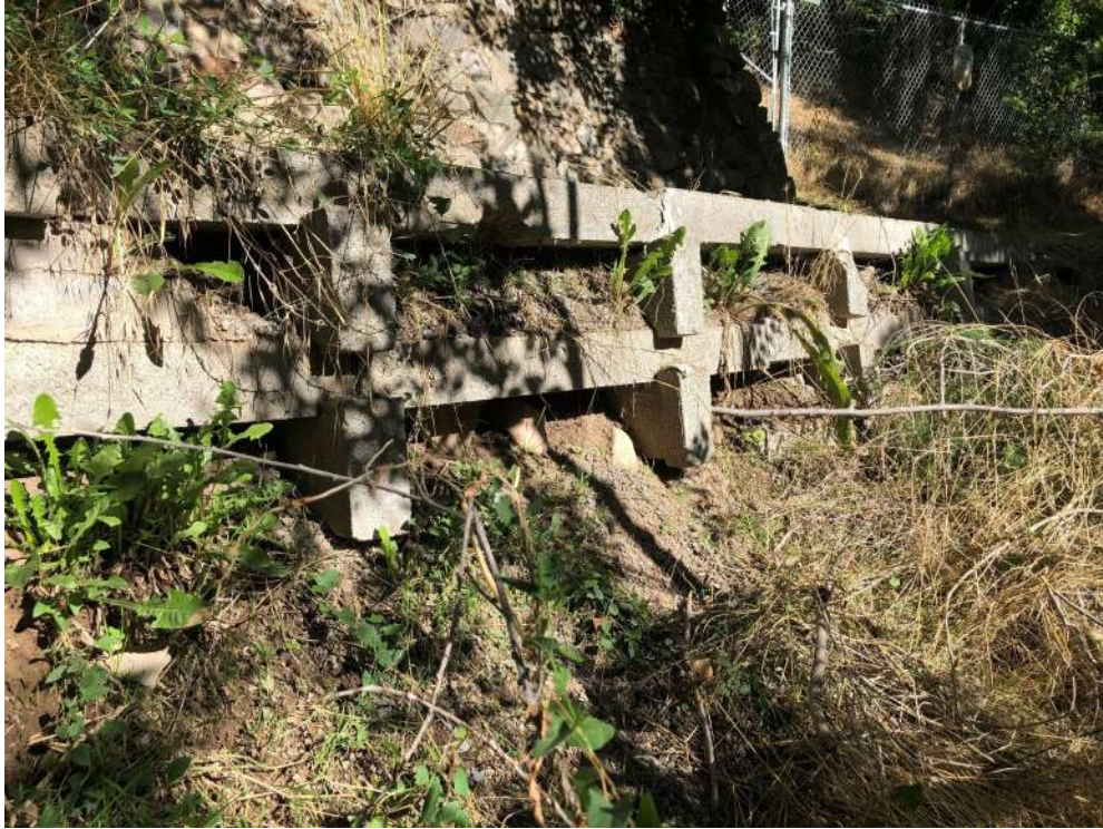
Photograph 7 - Crib wall on west side of creek has experienced erosion and undercutting.
