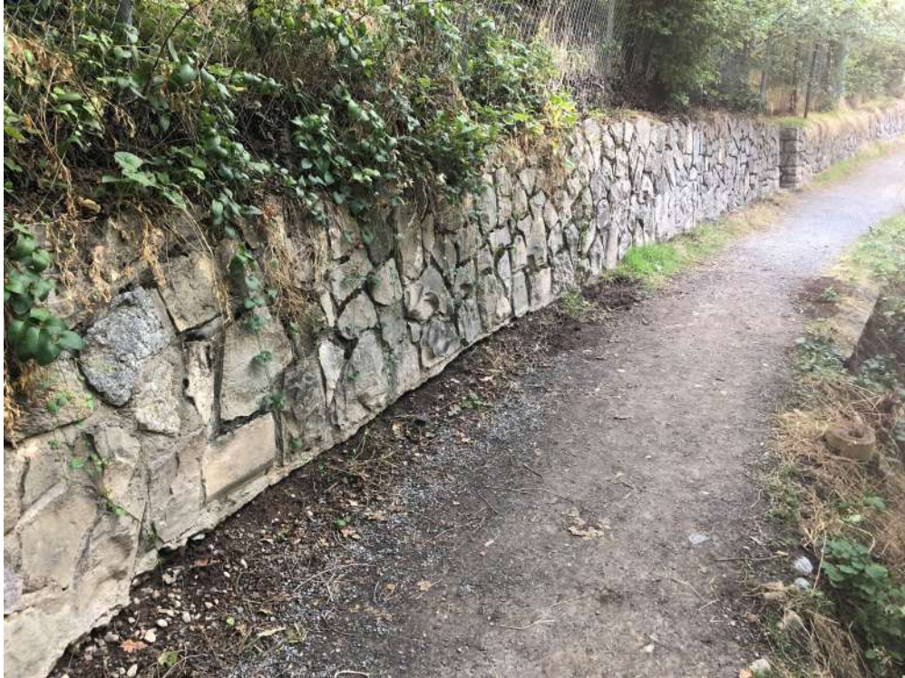
Photograph 6 - Ground at toe of wall appears lower than base rock.
