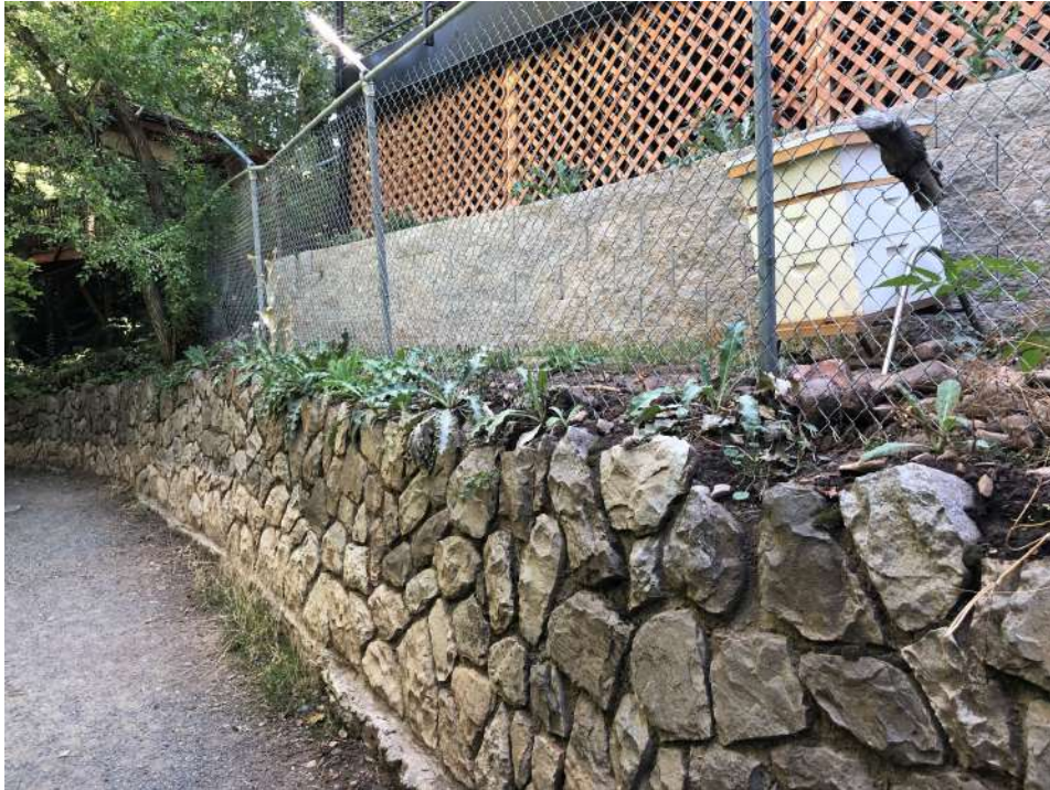
Photograph 13 - Area on the east side of creek where structures have been placed near the top of the wall. Also shown wall foundation exposed at the toe.
