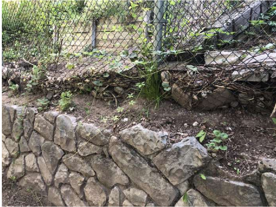
Photo #9 – Chainlink fences are collecting debris from runoff water and are retaining soil.
