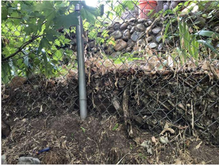
Photo #7 – Chainlink fences are collecting debris from runoff water and are retaining soil.
