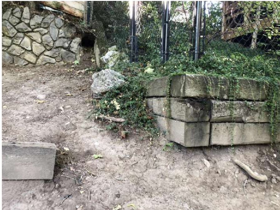
Photo #10 – Image of drainage from neighboring property owners and runoff from sprinklers causing the soil to erode and undermine the existing retaining wall structures.
