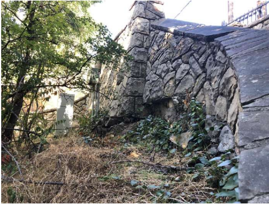
Photo #17 – The existing wall is being undermined and the toe needs to be covered with structural fill.
