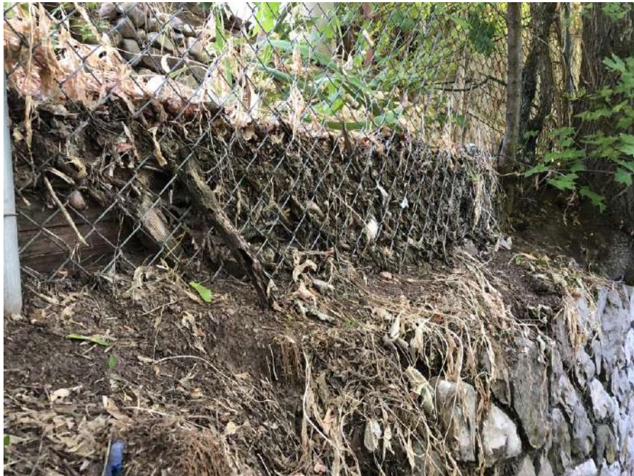
Photo #8 – Chainlink fences are collecting debris from runoff water and are retaining soil.
