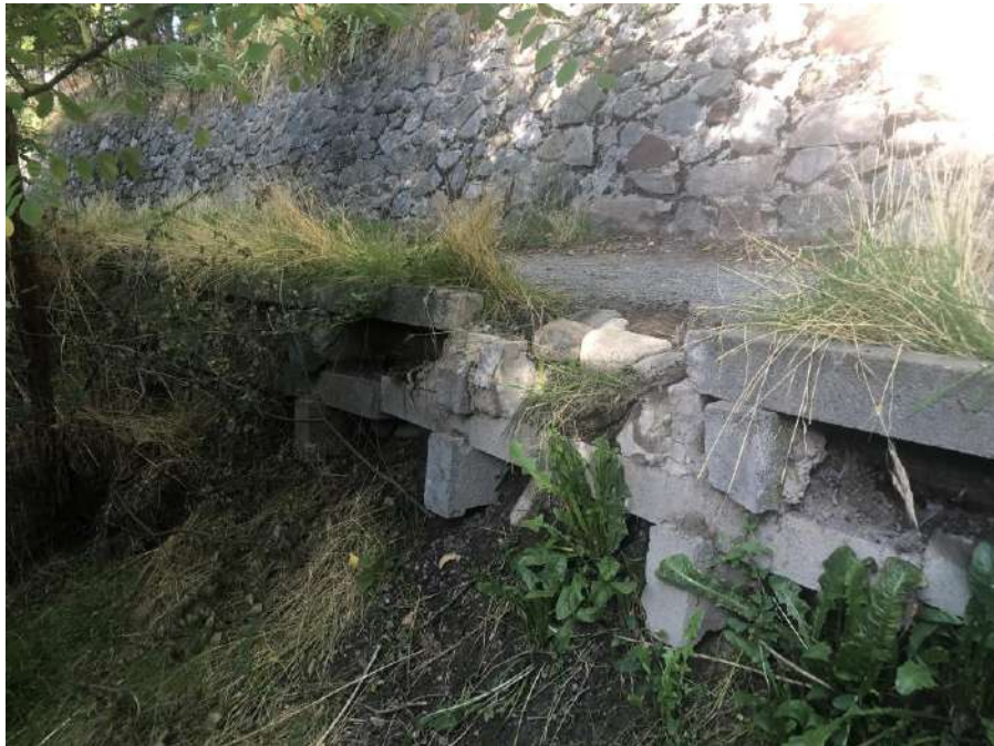
Photo #2 – erosion on the trail due to runoff and sprinklers has cause the crib walls to fail in several locations.
