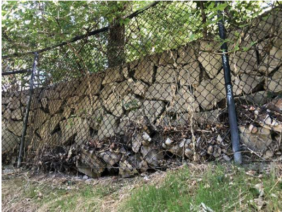
Photo #16 – There is a retaining wall built above the original rock wall that has large rocks caught in the fence. This wall is an example of neighbors building structures above the existing walls and creating additional loads on the existing structure.
