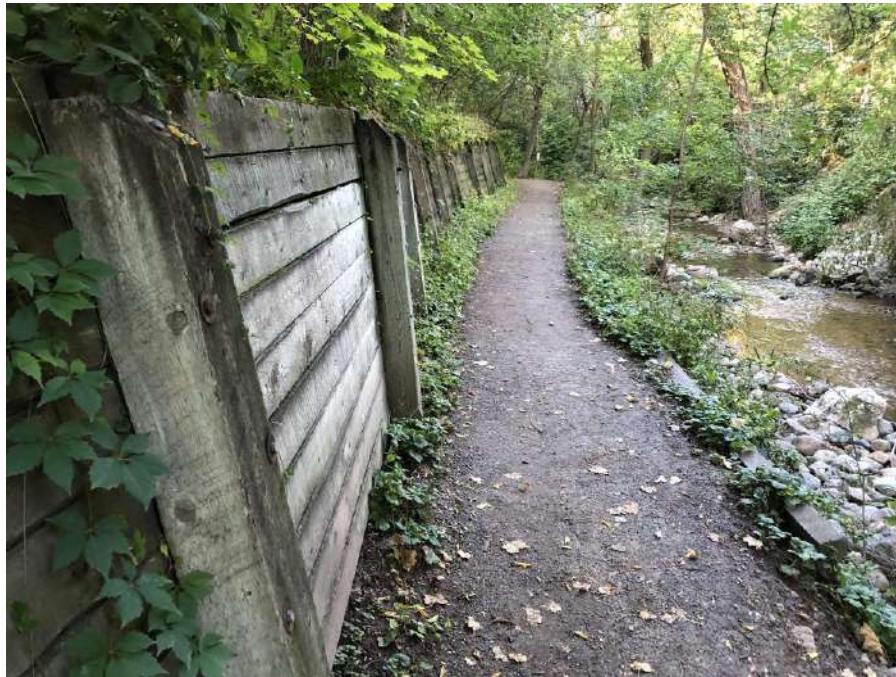
Photo #3 – Runoff from adjacent property owners' gutters is causing the wall to bulge and fail
