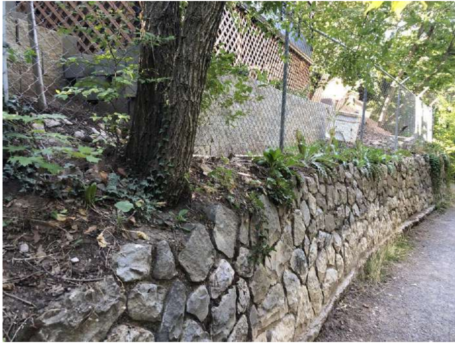
Photo #13 – Example of neighboring property owners building structures above existing rock walls. Trees that occur adjacent to the wall should be removed and the structural fill should be used to backfill over the toe of the existing rock wall.
