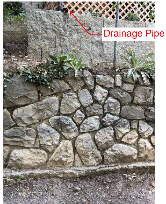
Photo #6 – Image of drainage pipe from neighboring property owners, example of adjacent structures encroaching on the existing rock walls, and example of toe of retaining wall being undermined.
