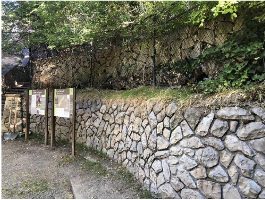
Photo #15 – There is a retaining wall built above the original rock wall that has large rocks caught in the fence. This wall is an example of neighbors building structures above the existing walls and creating additional loads on the existing structure.
