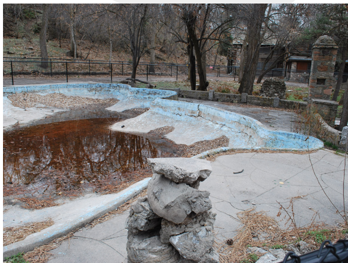
Figure 3-10. View looking southwest across the pool area.
