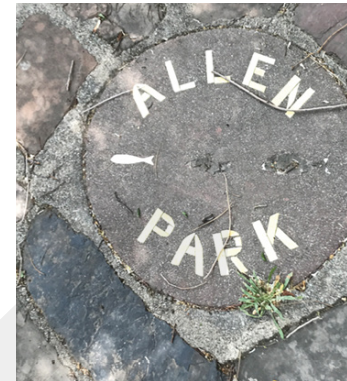
Unit paving & artwork concrete
