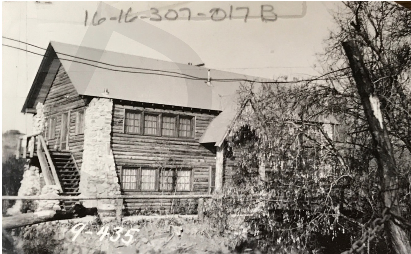
Figure 2-19. Ye Olde George Albert apartments, c. 1939. (H-3-H)
