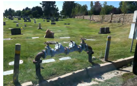
Irrigation Equipment - RPZ Source: Cemetery Planning Team
