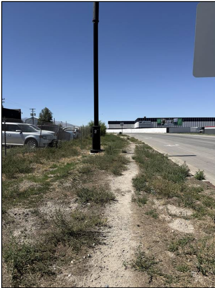
Existing Sidewalk on 400 S
