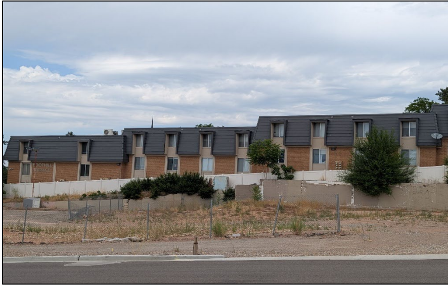
Adjacent property to North
