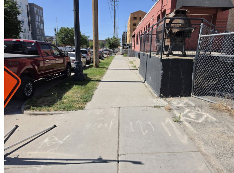
Existing sidewalk along 400 W looking south
