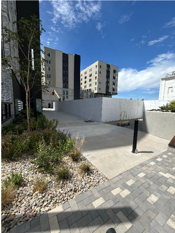
Portion of mid-block walkway north of interior park
