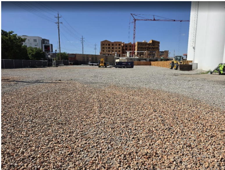
View from north property line looking south
