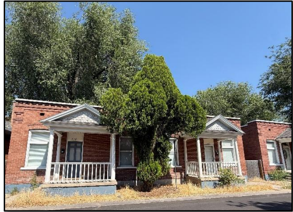
Quadplex on Denver Street
