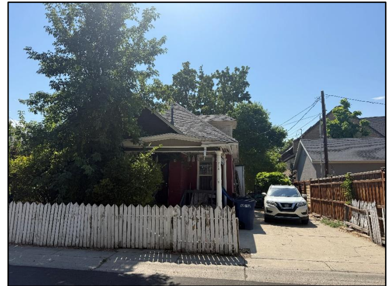
Adjacent Property to West of Subject Property
