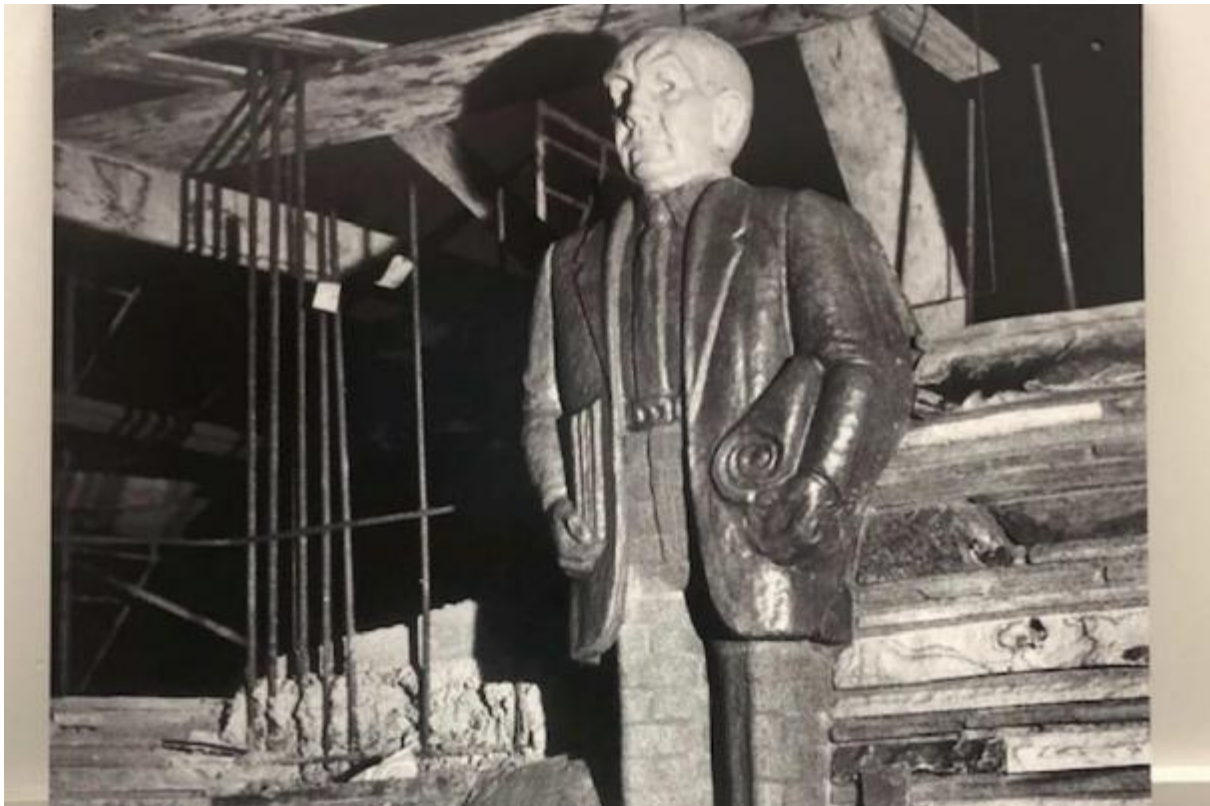
Figure 11 Constructing The Monument to the Trade. Thomas Battersby Child Papers, 1909–2002.
