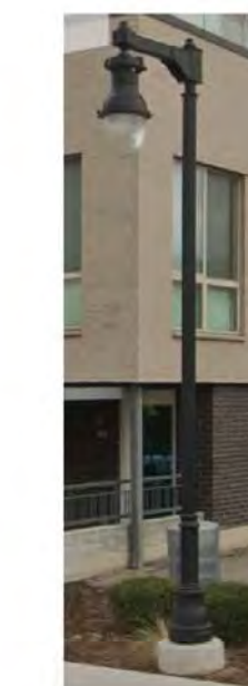
G PEDESTRIAN "ACORN" LIGHT POLE • SINGLE HEAD ACORN LIGHT TO MATCH SUGARHOUSE STANDARD
