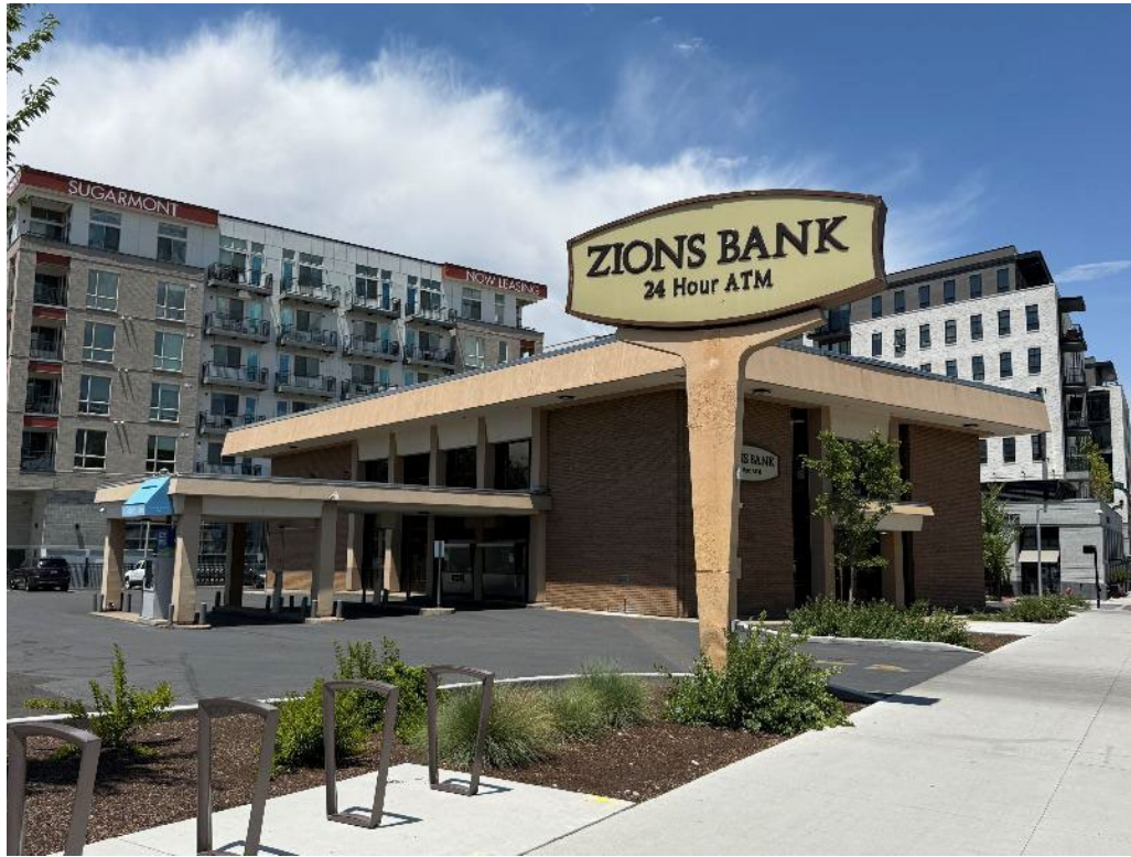
Existing Zions Bank building, facing northwest
