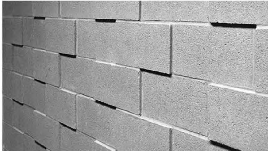
OFFSET GROUND FACE CMU COLOR: TBD COMMENTS: ALTERNATING OFFSET TYPE MARK: EX-MU2
