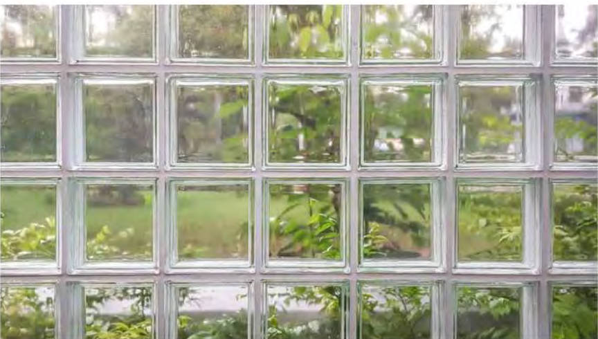
GLASS BLOCK COLOR: CLEAR COMMENTS: STACKED BOND TYPE MARK: EX-GB
