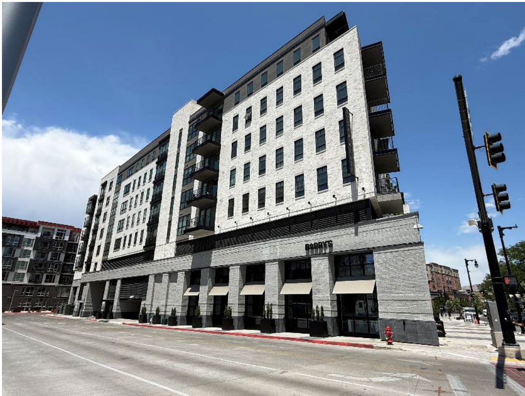
Sugar Alley building to the north of the subject property, facing northwest
