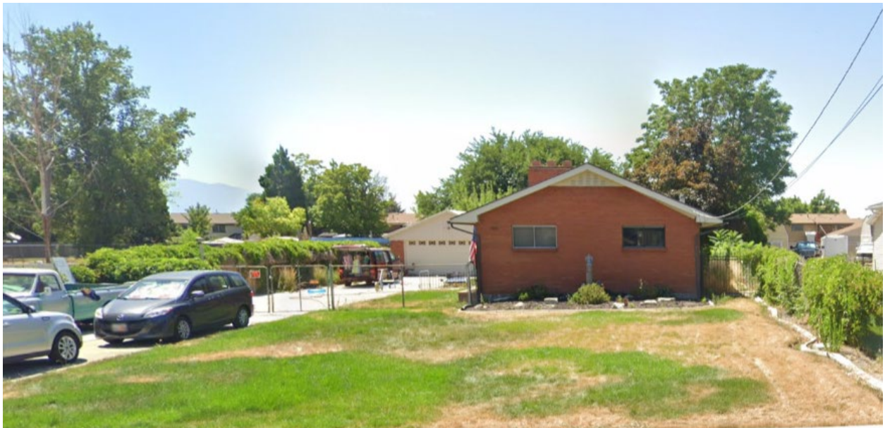
1395 W Van Buren. The home and the accessory structure are currently being demolished.
