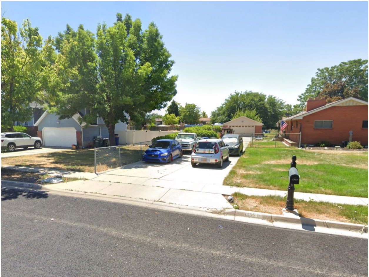
Subject properties. 1379 W Van Buren is on the left and is proposed to remain. The brick home is currently being demolished.
