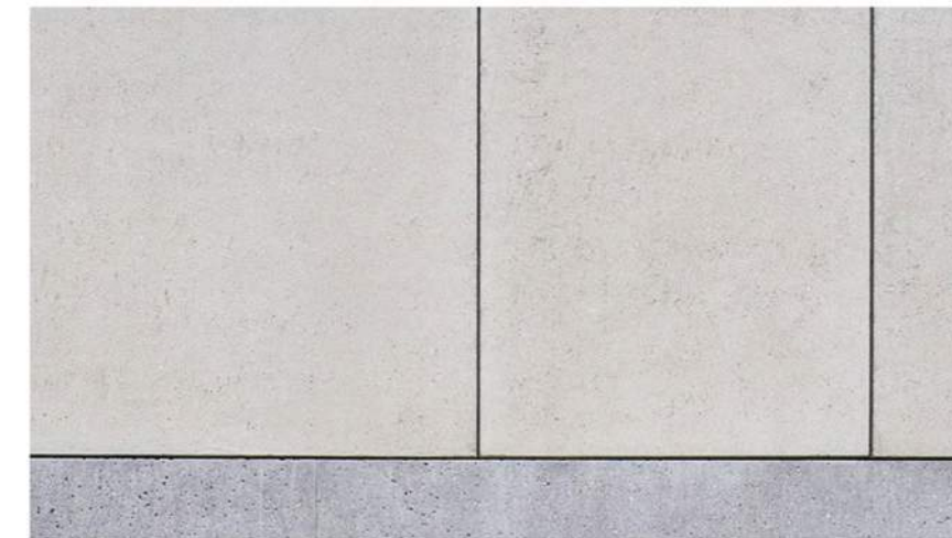
CAST STONE VENEER COLOR: TBD COMMENTS: MODULAR PRECAST VENEER PANEL TYPE MARK: EX-CSV
