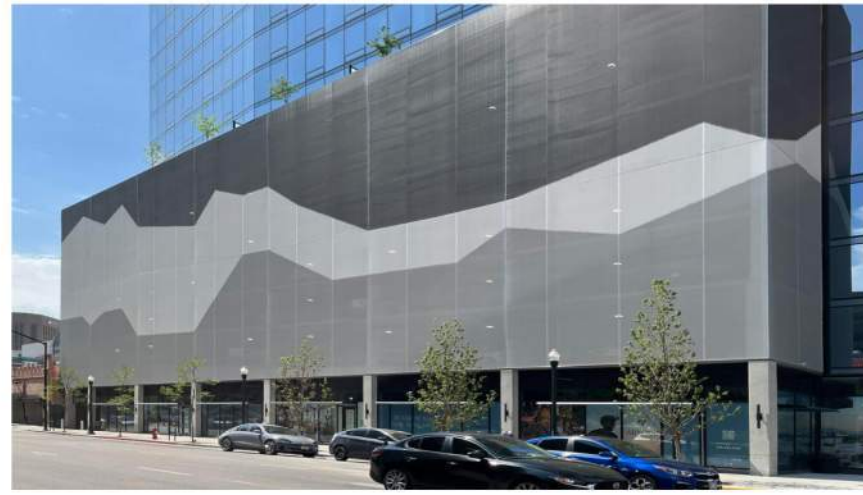
DECORATIVE SCREENING PANEL (FLEXFACADE) COLOR: CUSTOM GRAPHIC MURAL COMMENTS: 34% OPEN TYPE MARK: EX-DSP
