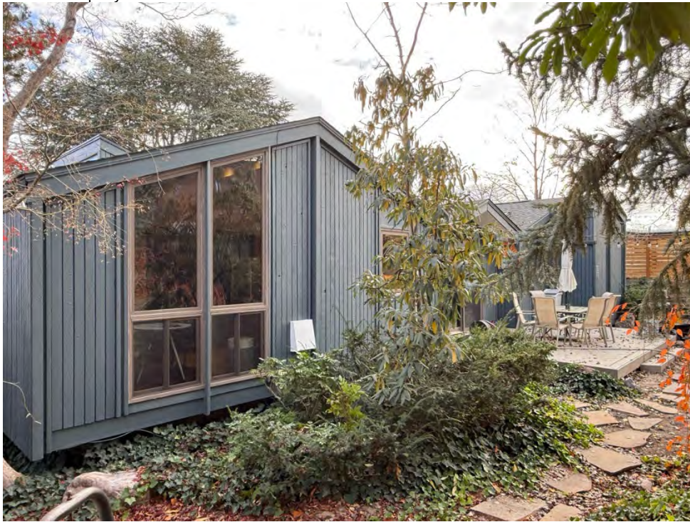
Photograph 8. Exterior, north façade. Camera facing southwest.
