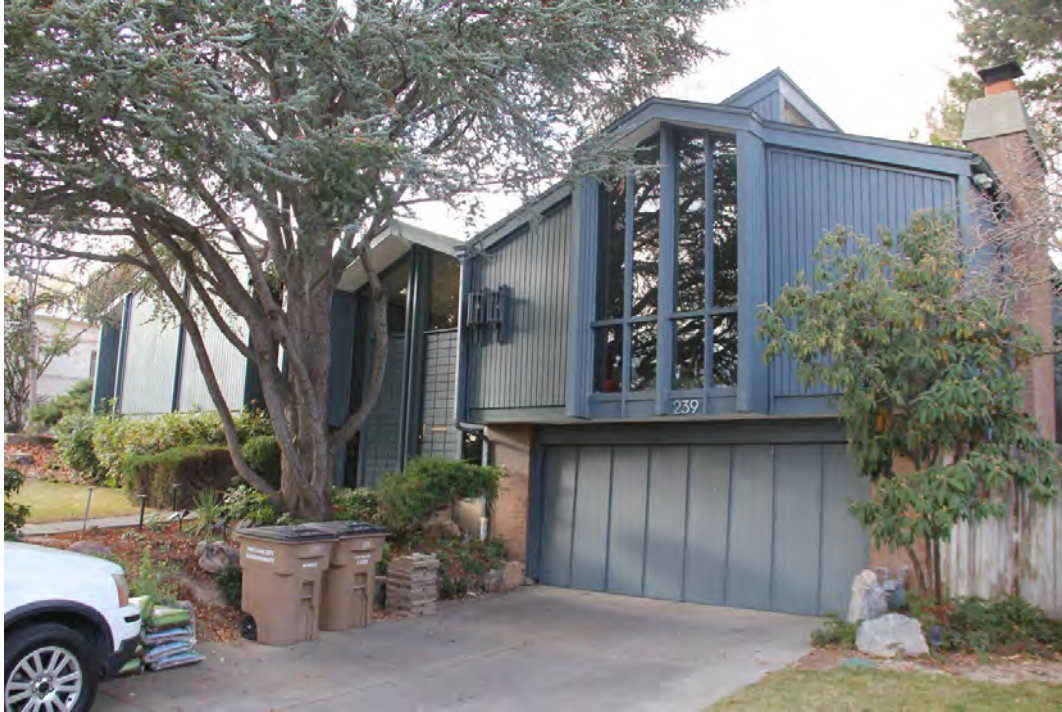
Photograph 1. Exterior, south (main) façade. Camera facing northwest.
