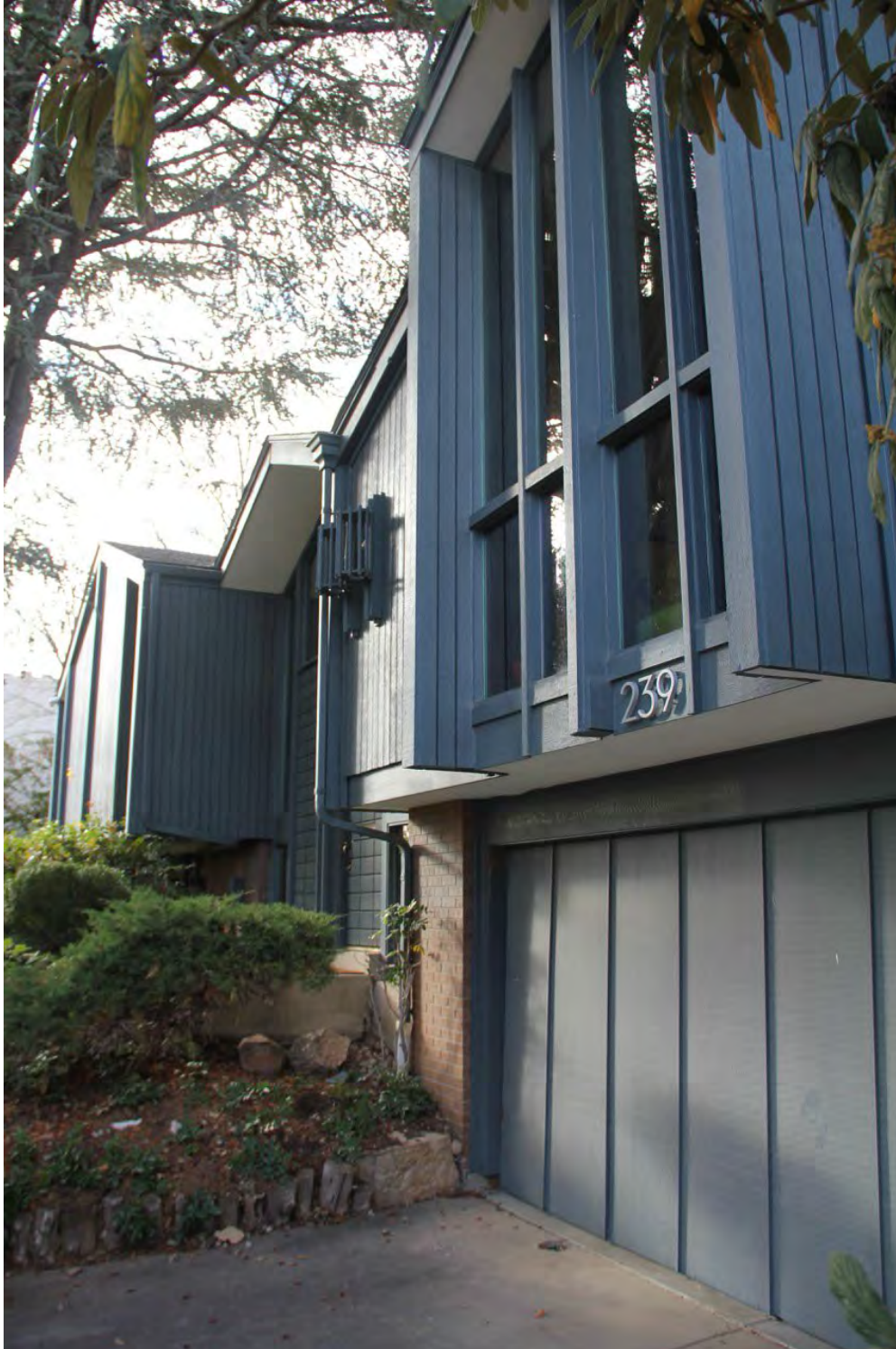
Photograph 12. Exterior, south (main) façade showing details of garage, and exterior siding. Camera facing west.
