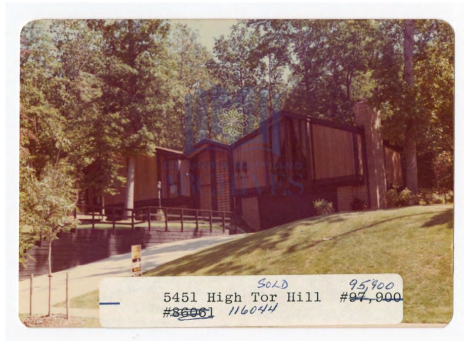
Figure 6. Photograph of 5451 High Tor Hill, Columbia, Maryland 21045, taken c. 1975. This house was built c. 1973. Source: Columbia Maryland Archives.
