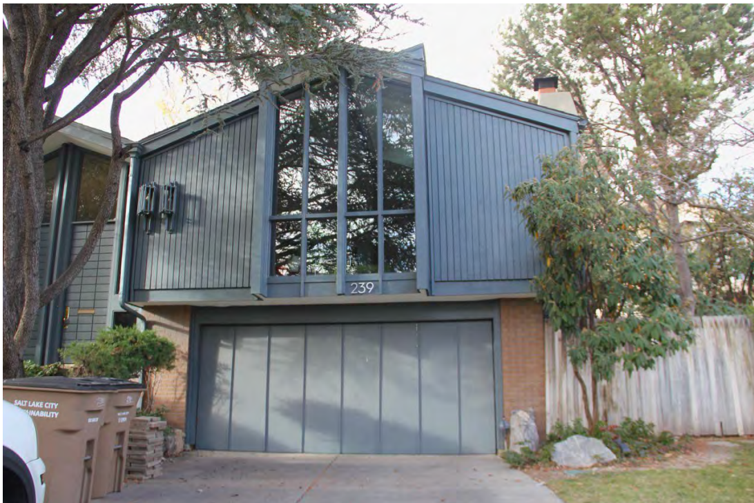
Photograph 4. Exterior, south (main) façade showing details of the trapezoidal windows. Camera facing north.
