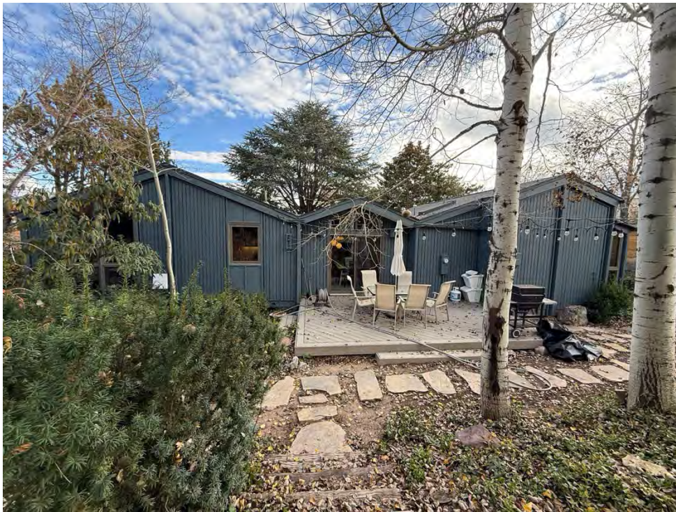
Photograph 9. Exterior, north façade. Camera facing south.
