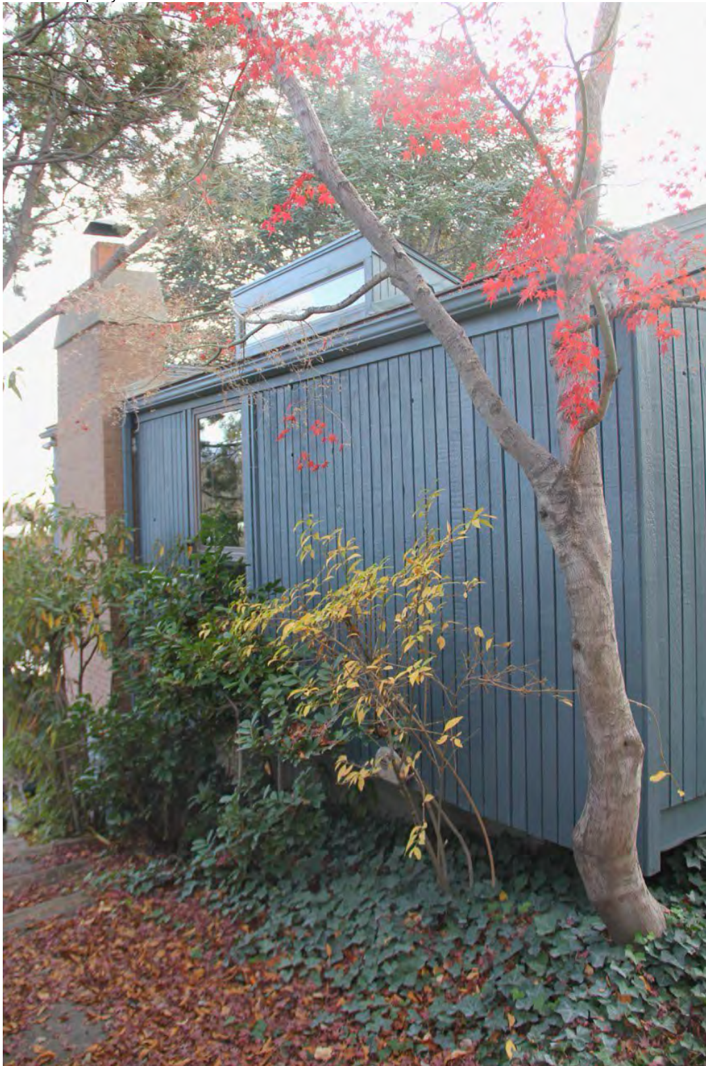
Photograph 7. Exterior, east façade. Camera facing southwest.
