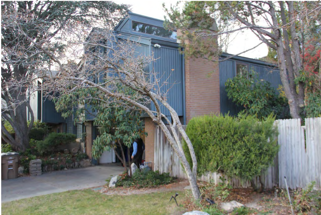
Photograph 5. Exterior, corner of south (main) and east façade. Camera facing northwest.
