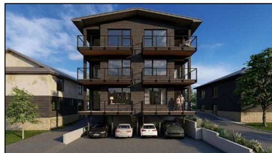
Rear elevation (approx. 44’ tall) of the new construction – Additional building height is being requested
