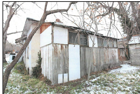
Rear addition to be removed
