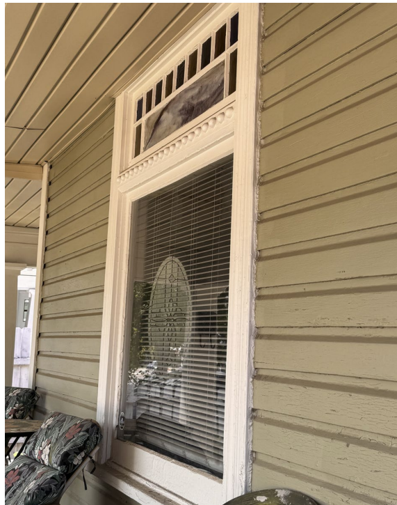
Original wood windows on front and north side of subject dwelling
