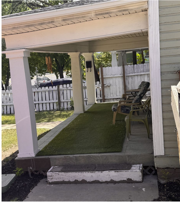
View of porch from the North
