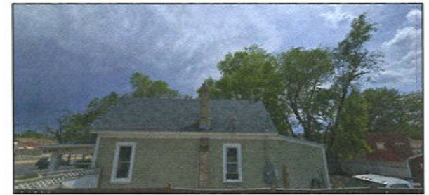
EXISTING LOCATION BUILDING NORTH ELEVATION
