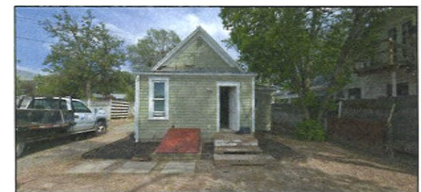
EXISTING LOCATION BUILDING WEST ELEVATION
