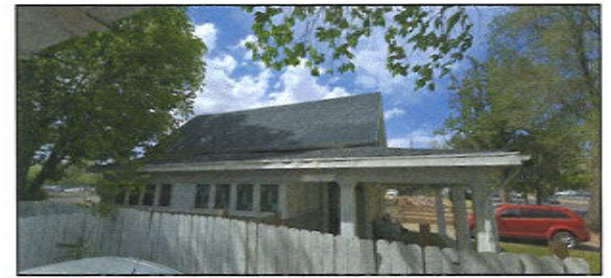
EXISTING LOCATION BUILDING SOUTH ELEVATION
