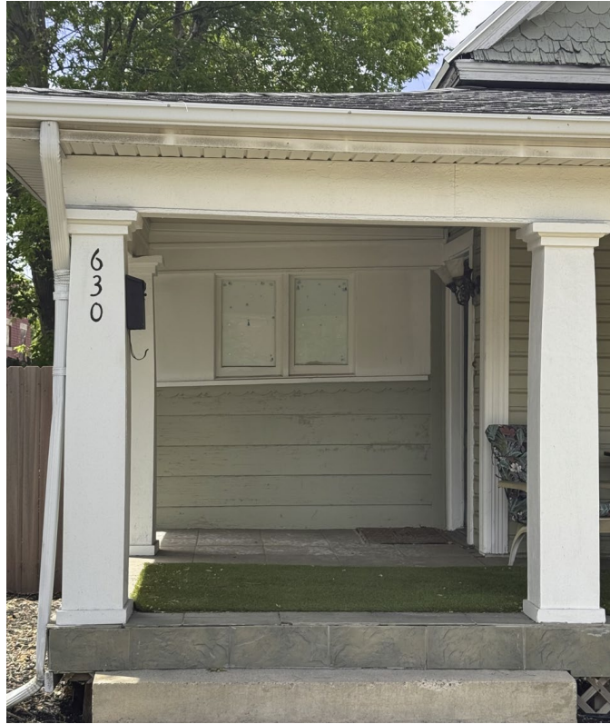
View of the south side of the porch -looking from 700 East
