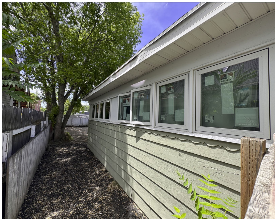
View of the south side of the dwelling -most likely an older addition- showing newly replaced windows and the scalloped wooden trim molding above the siding
