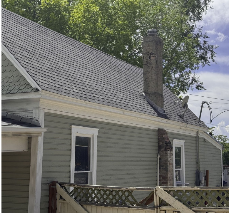
View of the North side of the dwelling – brick chimney
