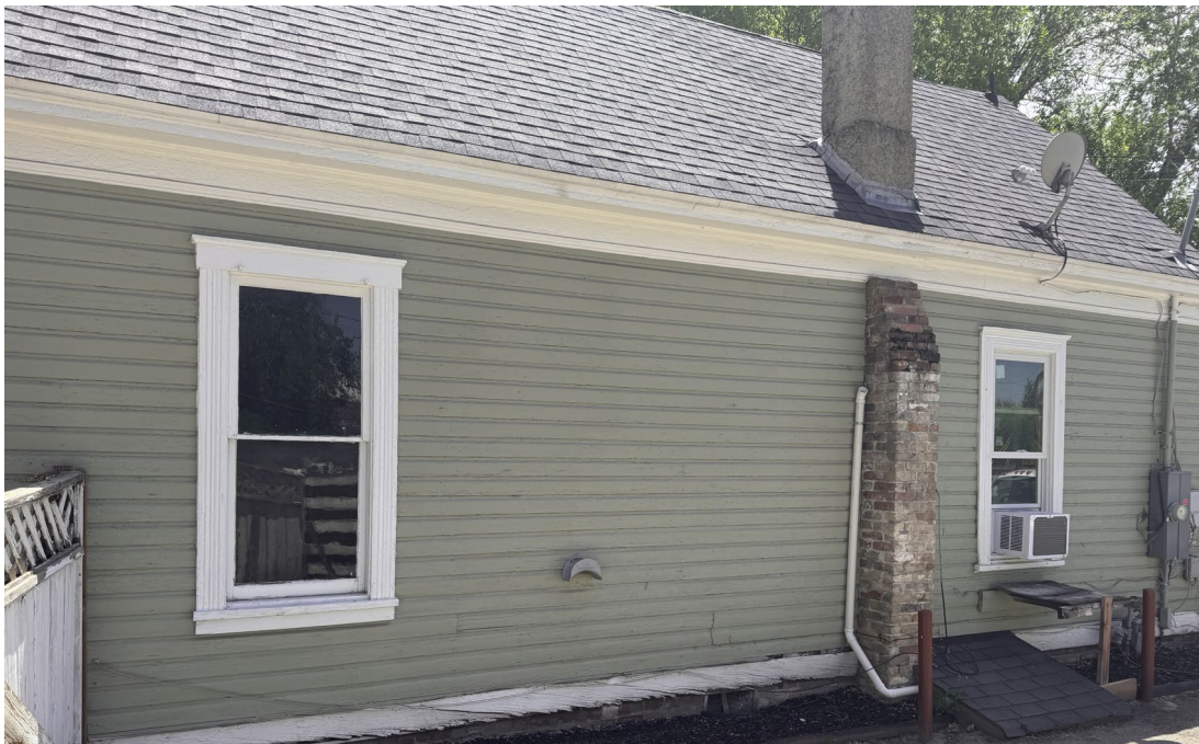
View of the North side of the dwelling – showing the original wood windows and horizontal wood cladding siding with a scooped profile at the top
