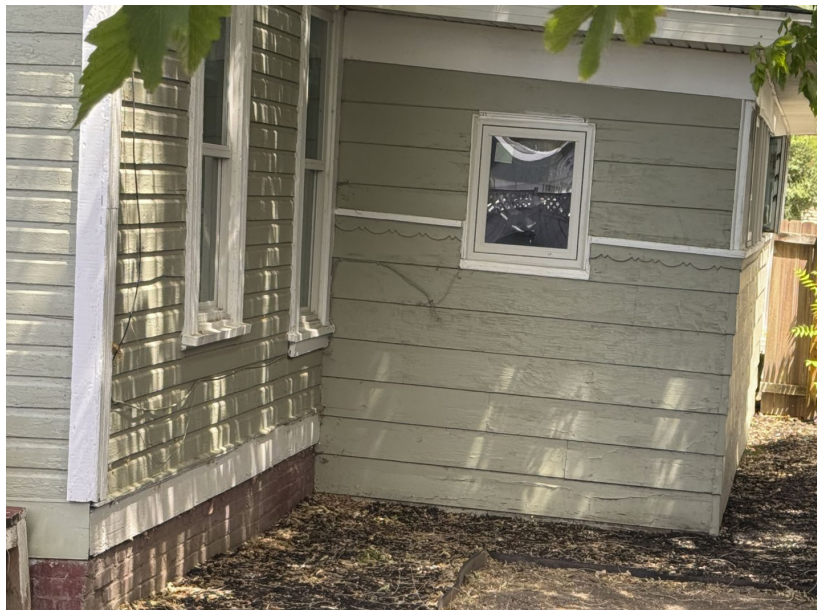
View of the south side of the dwelling – likely a later addition to the dwelling- shows Wider wood lap clad siding
