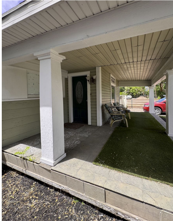
View to the northwest -showing the front door and covered porch area
