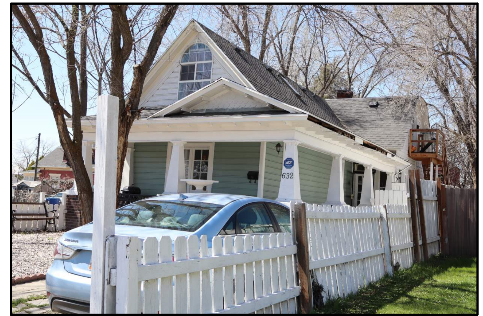
EXISTING LOCATION BUILDING #5 NORTH ELEVATION
