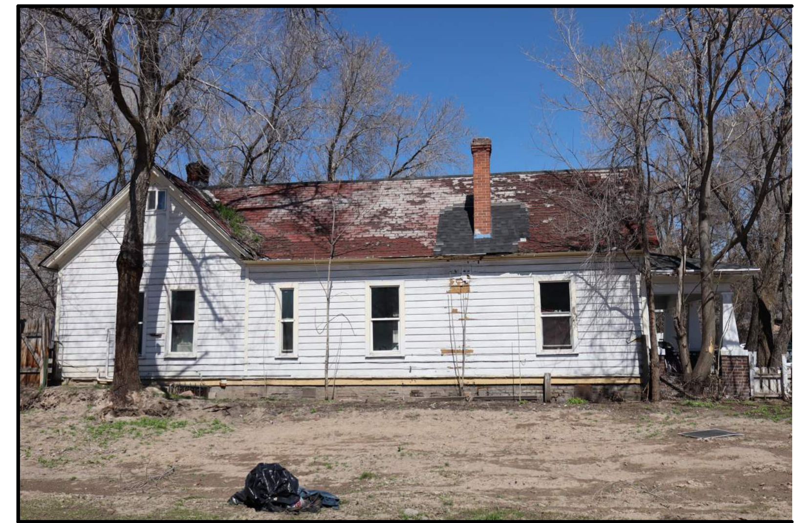
EXISTING LOCATION BUILDING #5 SOUTH ELEVATION
