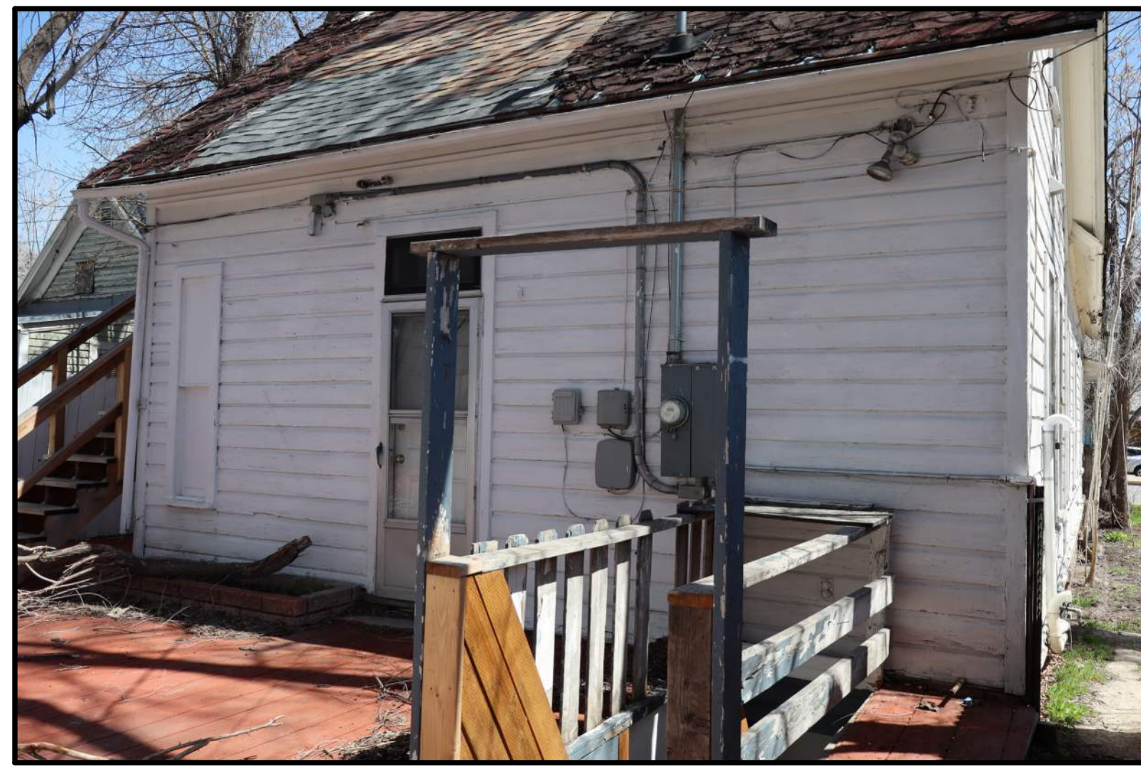
EXISTING LOCATION BUILDING #5 WEST ELEVATION
