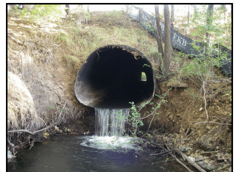
Top left: Debris and sediment accumulation at culvert inlet. Top right: Erosion at storm drain outfall. Bottom left: Invasive vines on streambank. Bottom right: Scour at culvert outlet.
