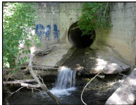
Top left: Invasive vines on streambank. Top right: Debris and sediment accumulation at culvert inlet. Bottom left: Scour at culvert outlet. Bottom right: Erosion at storm drain outfall.
