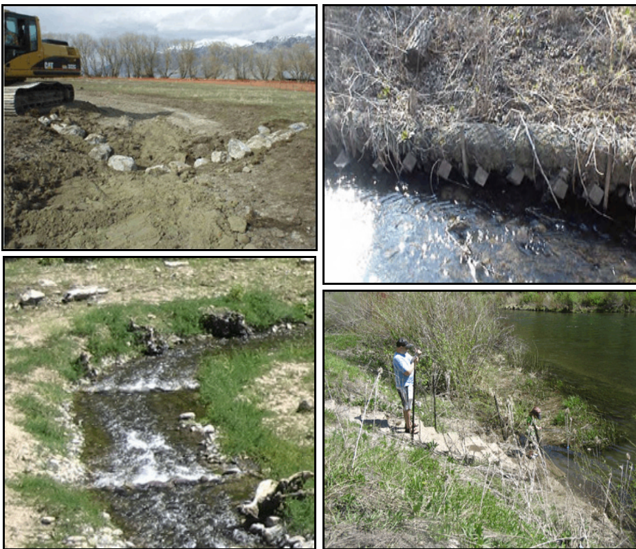
Figure 4.6. Photographs of grade-control, bank-stabilization, and access-control techniques. Top left: construction of a vortex rock weir. Top right: A-jacks toe protection (image from Schueler and Brown 2004). Bottom left: downstream view of two vortex rock weir structures. Bottom right: steps that provide stabilized stream access.
