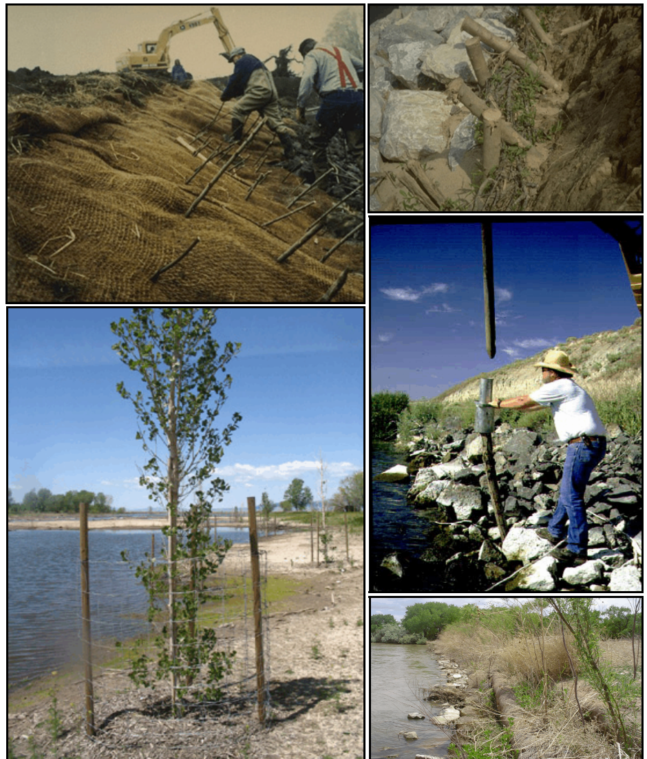
Figure 4.4. Photographs of revegetation and biotechnical slope-stabilization techniques. Top left: erosion-control blanket and live stakes (image from FISRWG 1998). Top right: live pole plantings (image from FISRWG 1998). Bottom left: containerized cottonwood ( Populus sp.) planting protected from herbivory with wire mesh cage. Middle right: installation of live plant posts to create vegetated rock revetment (image from NRCS 2007). Bottom right: vegetated soil lifts with live plant stakes and rock toe protection.
