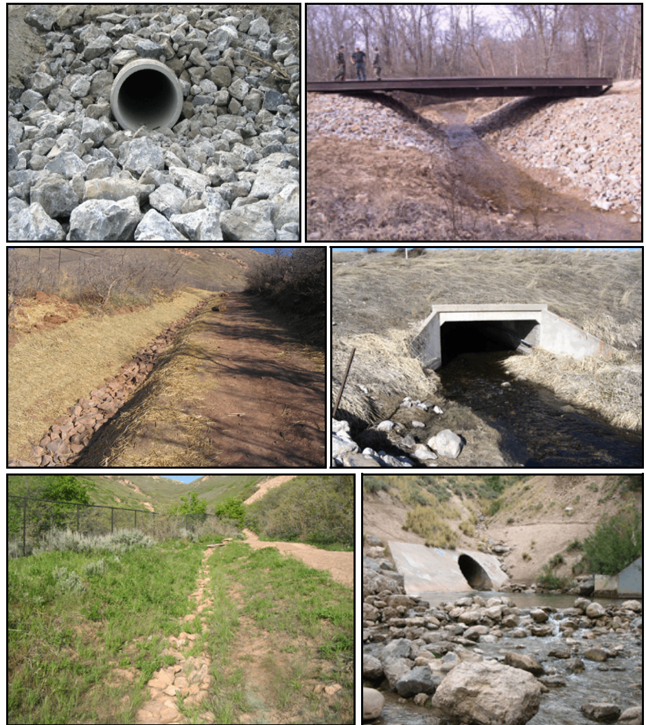
Figure 4.5. Photographs of outlet protection and stream crossing techniques. Top left: rock outlet protection. Top right: stream crossing using a bridge made from a recycled railroad flatcar. Middle left: vegetated rock-lined swale immediately following construction. Middle right: stream crossing using an open-bottom box culvert. Bottom left: vegetated rock-lined swale in second growing season. Bottom right: tailwater pool at culvert outlet.
