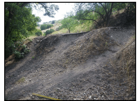
Top left: Steep bare slope adjacent to Bonneville Boulevard in reach LCC_R01A. Note trees, grass, and large rocks at base of slope indicating toe stability. Top right: Rill erosion below pipe outfalls. Bottom left: Rill erosion where road runoff concentrates at gabion/natural bank interface. Bottom right: Bare bank and compacted soil associated with heavy recreational foot traffic.
