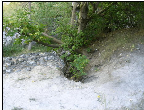
Top left: Steep bare slope adjacent to Bonneville Boulevard in reach LCC_R01A. Note trees, grass, and large rocks at base of slope indicating toe stability. Top right: Rill erosion below pipe outfalls. Bottom left: Rill erosion where road runoff concentrates at gabion/natural bank interface. Bottom right: Bare bank and compacted soil associated with heavy recreational foot traffic.
