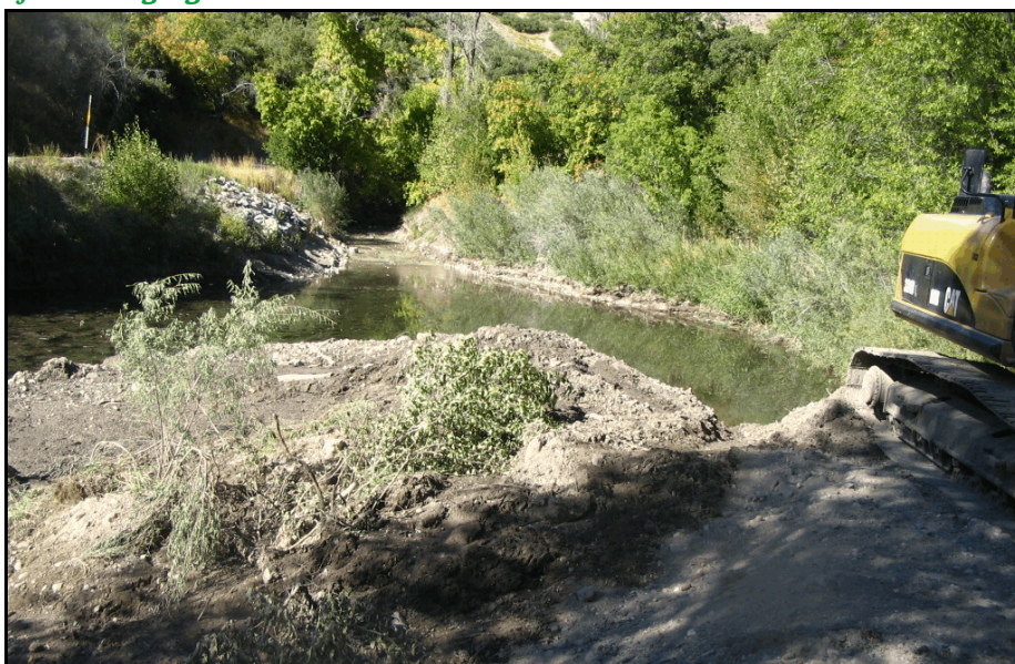
Below: City Creek debris basin above Bonneville Boulevard shortly after dredging.
