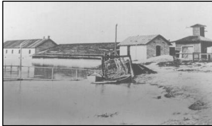
The Utah Lake Pumping Plant, owned by the Associated Canals, is located at the outlet of the lake. In 1907 this was the largest pumping plant in the United States, capable of pumping 700 cfs or 452 mgd.
