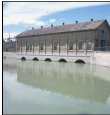
Intake view of the Utah Lake Pumping Plant as viewed in 1989.
