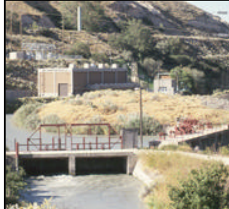
The Turner Dam was constructed in 1914, and replaced the "Old Dam." On the left, water is diverted to the East Jordan Canal and on the right, water is diverted to the Utah and Salt Lake Canal. In the background is the Salt Lake County Water Conservancy District Pump Plant, and behind that facility is the Metropolitan Water District of Salt Lake City Pump Plant. The Salt Lake County Conservancy Pumping Plant provides exchange water to the Provo Reservoir Canal and the Metropolitan Water District exchange water to the Utah Lake Distribution Canal- both on the west side of the Jordan River.
