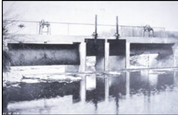
The Joint Dam located about one mile below the Turner Dam on the Jordan River is the diversion point for the Jordan & Salt Lake City Canal and the South Jordan Canal. This structure was replaced after the 1983 flood.
