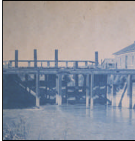
The "Old Dam" located at the Jordan Narrows was built by the County in 1872. Under the same project the County began construction of the Utah and Salt Lake Canal. The dam consisted of timber uprights set in cement, between which planks were inserted to raise water into the East Jordan and Utah and Salt Lake Canals.
