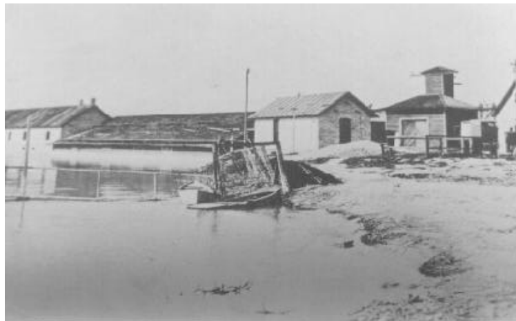
Utah Lake Pumping Plant as viewed in 1901. By 1907, the pump plant was the largest in the United States at 700 cfs.
