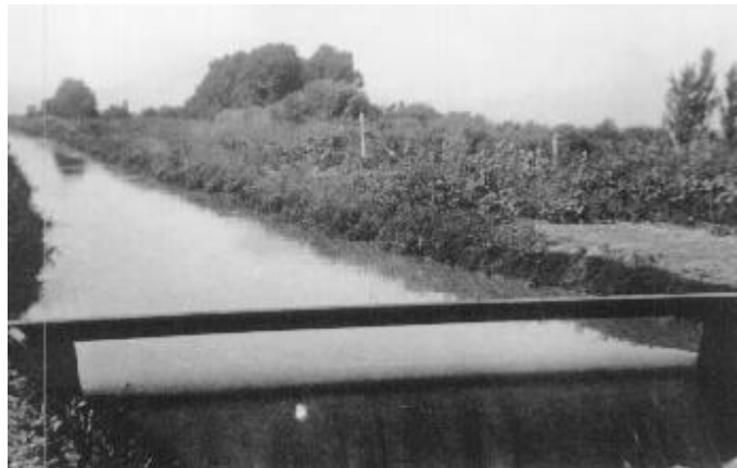
Jordan & Salt Lake Canal at 11 th East and 12 th South, looking south. Designed to carry 150 cfs, the Canal as viewed in 1900.
