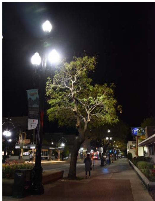
The historic acorn style lights currently used on the Downtown "Cactus" pole distribute a significant amount of light upward, contributing to increased light pollution and sky glow.
