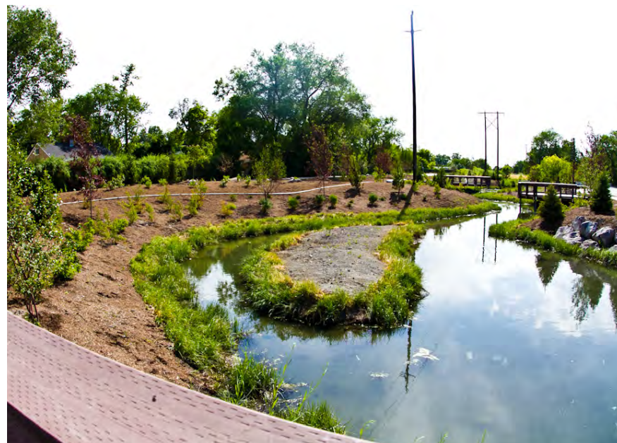
900 South Constructed Wetlands beautification improvements were made to the previously empty area between the 9 Line and 900 South west of 900 West in 2014
