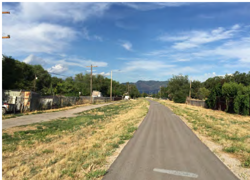
Existing 9 Line Trail a block east of Redwood Rd, looking east
