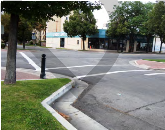
Bulb-out for on-street parking
