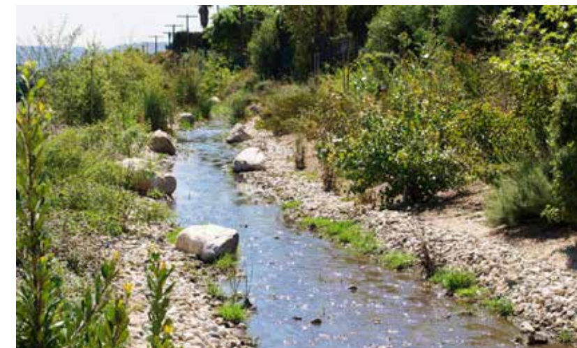
A naturalized section of the Tsunga Wash increases riparian habitat while providing stormwater infrastructure.
