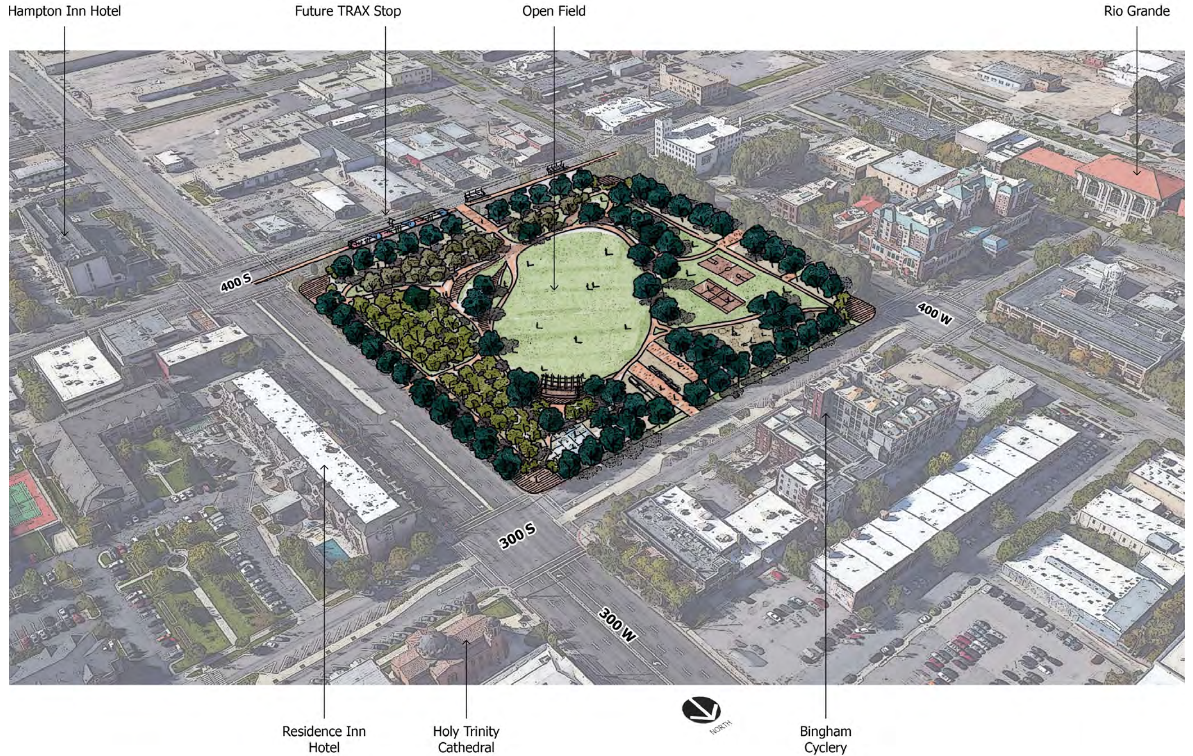
Overall Aerial View from North
