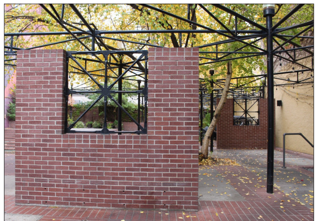
Brick and Steel Details at Dinwoodey Plaza (photo: Landmark Design)
