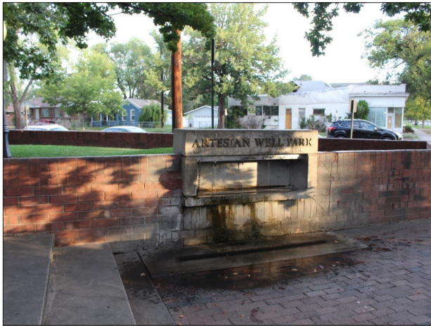
Spring at Artesian Well Pocket Park (photo: Landmark Design)
