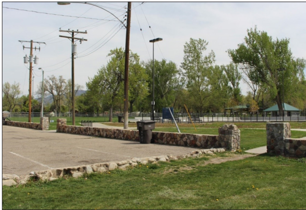
Walls and Sidewalk Entrance at Fairmont Park (photo: Landmark Design)
