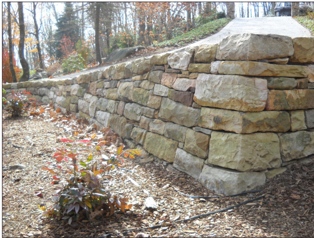
Example of Masonry Retaining Wall (photo: www.livingstonmasons.com )
