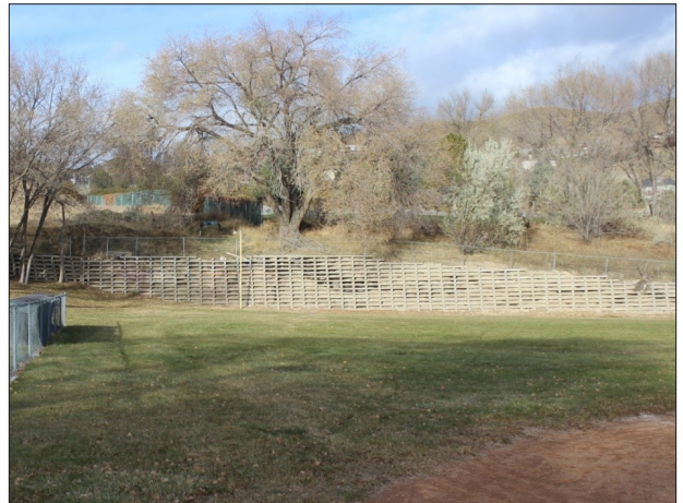
Timber Retaining Wall at Lindsey Gardens (photo: Landmark Design)
