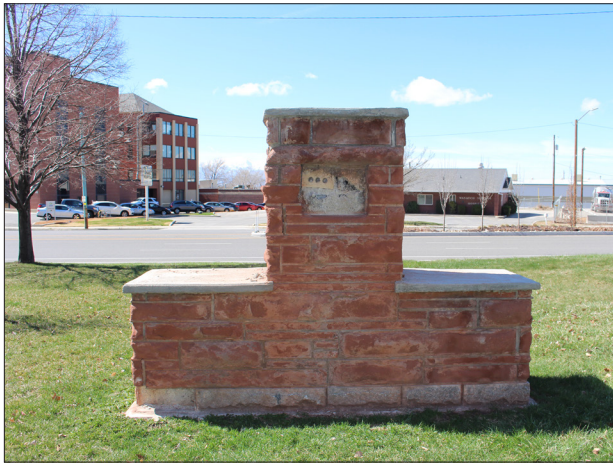
Stone and Concrete Monument at Warm Springs Park (photo: Landmark Design)
