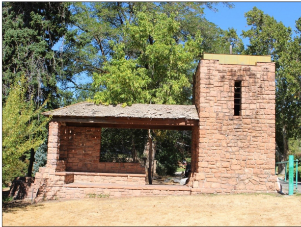
Restroom and Shelter at Bonneville Golf Course (photo: Landmark Design)
