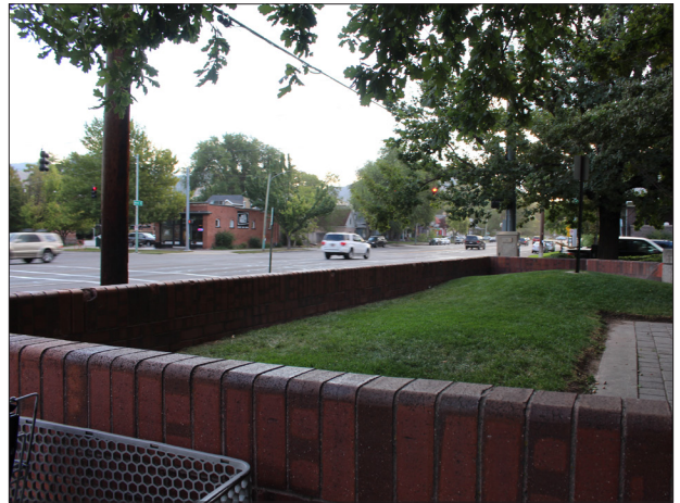
Wall and Grading at Artesian Well Park (photo: Landmark Design)
