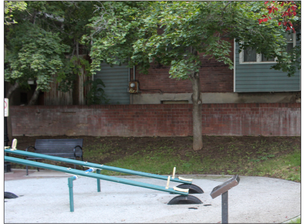
Masonry Retaining Wall at Silver Mini Park (photo: Landmark Design)
