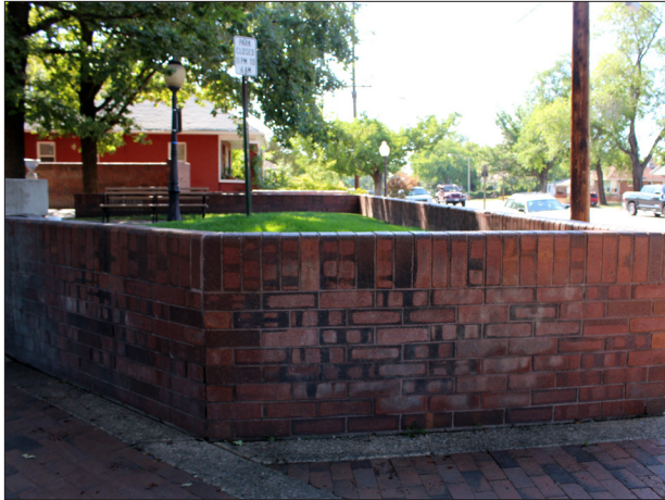
Brick Retaining Wall at Artesian Well Park (photo: Landmark Design)
