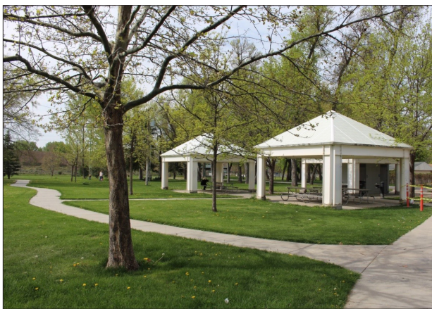
Small Pavilions at Riverside Park (photo: Landmark Design)
