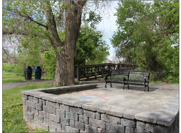
Masonry Retaining Wall at Riverside Park (photo: Landmark Design)
