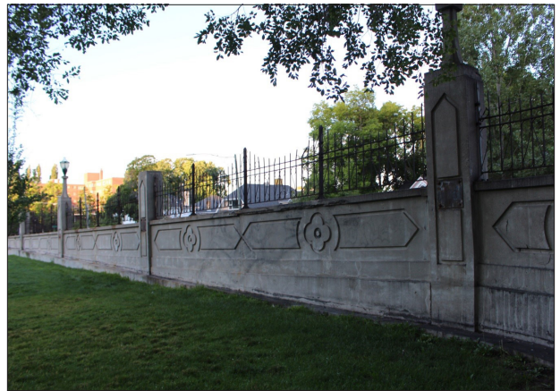
Concrete Wall at Reservoir Park (photo: Landmark Design)
