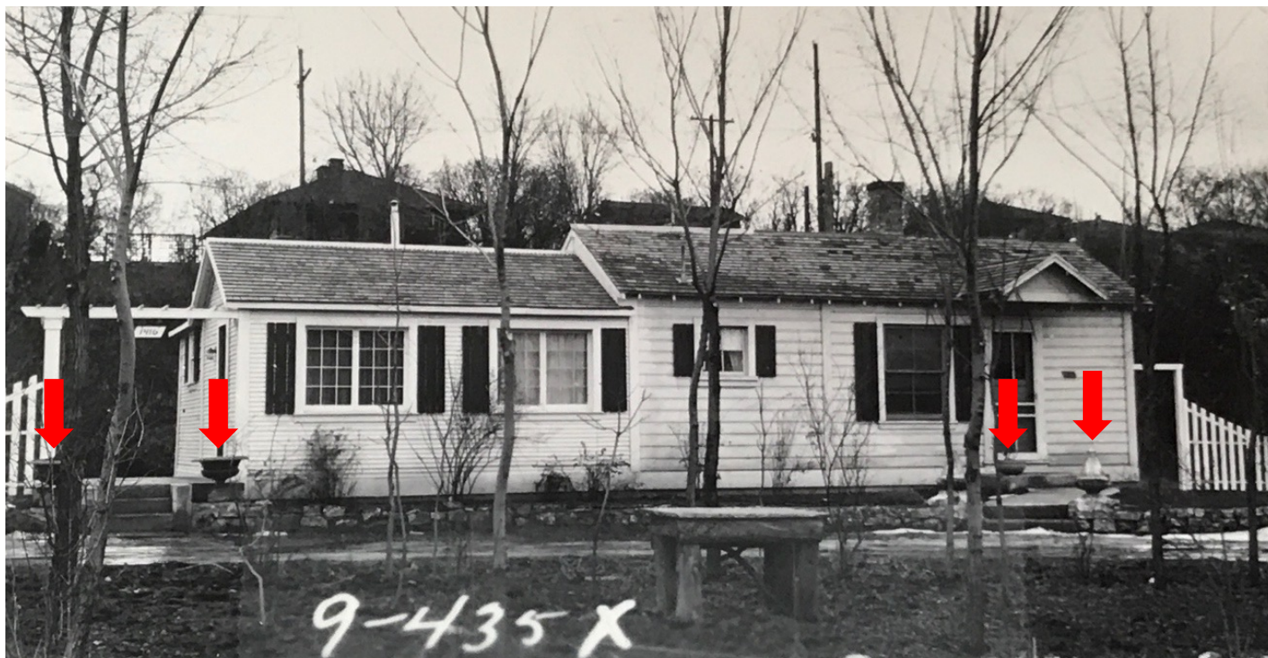
Figure 4-26. Ca. 1944 photo of the 1414-1416 East apartment with its gateway features.
