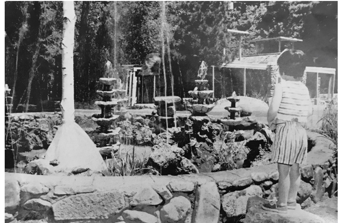
Figure 2-27. One of the constructed water features, "The elaborate fountain and many bird pens that compose... interesting Allen Park" in 1961. (H-4-V)
