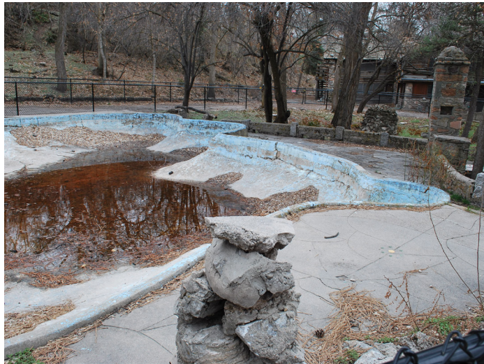
Figure 3-10. View looking southwest across the pool area.
