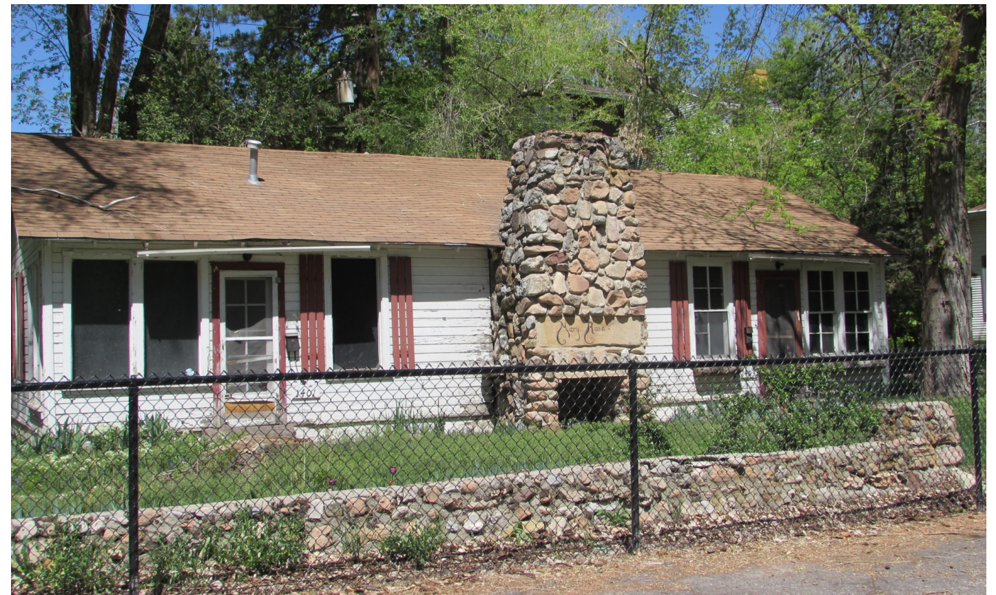
Figure 4-8. 2021 comparative photo of the Mary Rose cottage and its stone wall.
