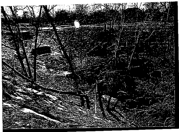
Photo 11. Stacked drains in the embankment at the southern end of the detention basin. Emigration Creek flows into the lowest drain in this picture. (A. Cannon)
