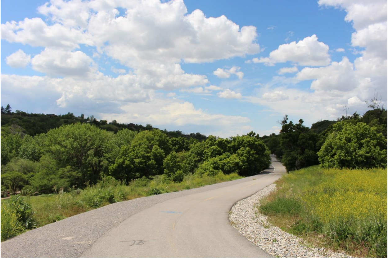
Fig. 63. View to the west of Parley’s Creek Corridor Trail located north of the “East Off-Leash Dog Area” (JoEllen Grandy, 5/27/16).
