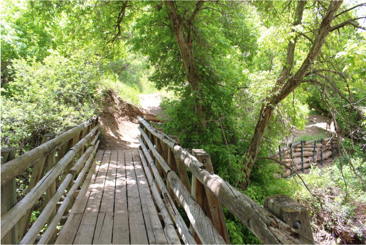
Fig. 83. View to the south of a footbridge located at the South Loop Trail trailhead access from the “Central Off-leash Dog Area”, approximately 0.52 miles from the main entrance into the park (JoEllen Grandy, 5/27/16).
