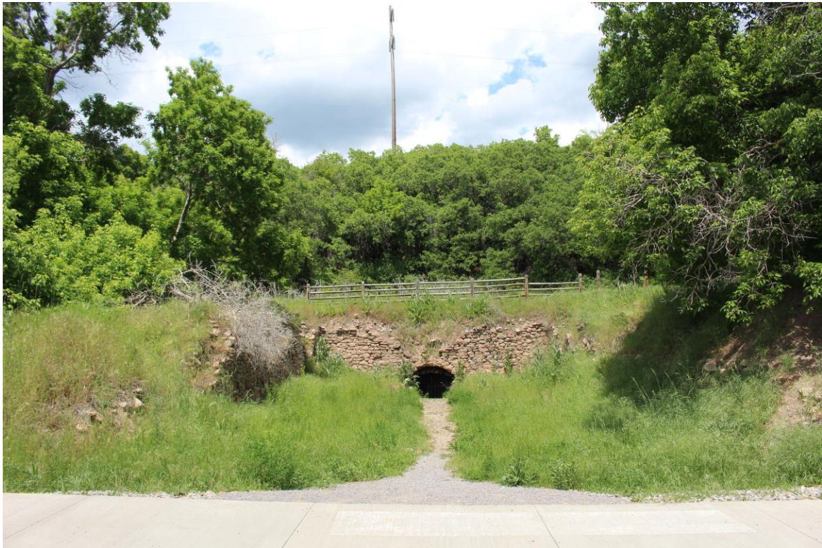
Fig. 73. View to the north of remnants of Dudler's Wine Cellar located on the northside of Parley's Creek Corridor Trail, immediately north of the large boulder monument (JoEllen Grandy, 5/27/16).
