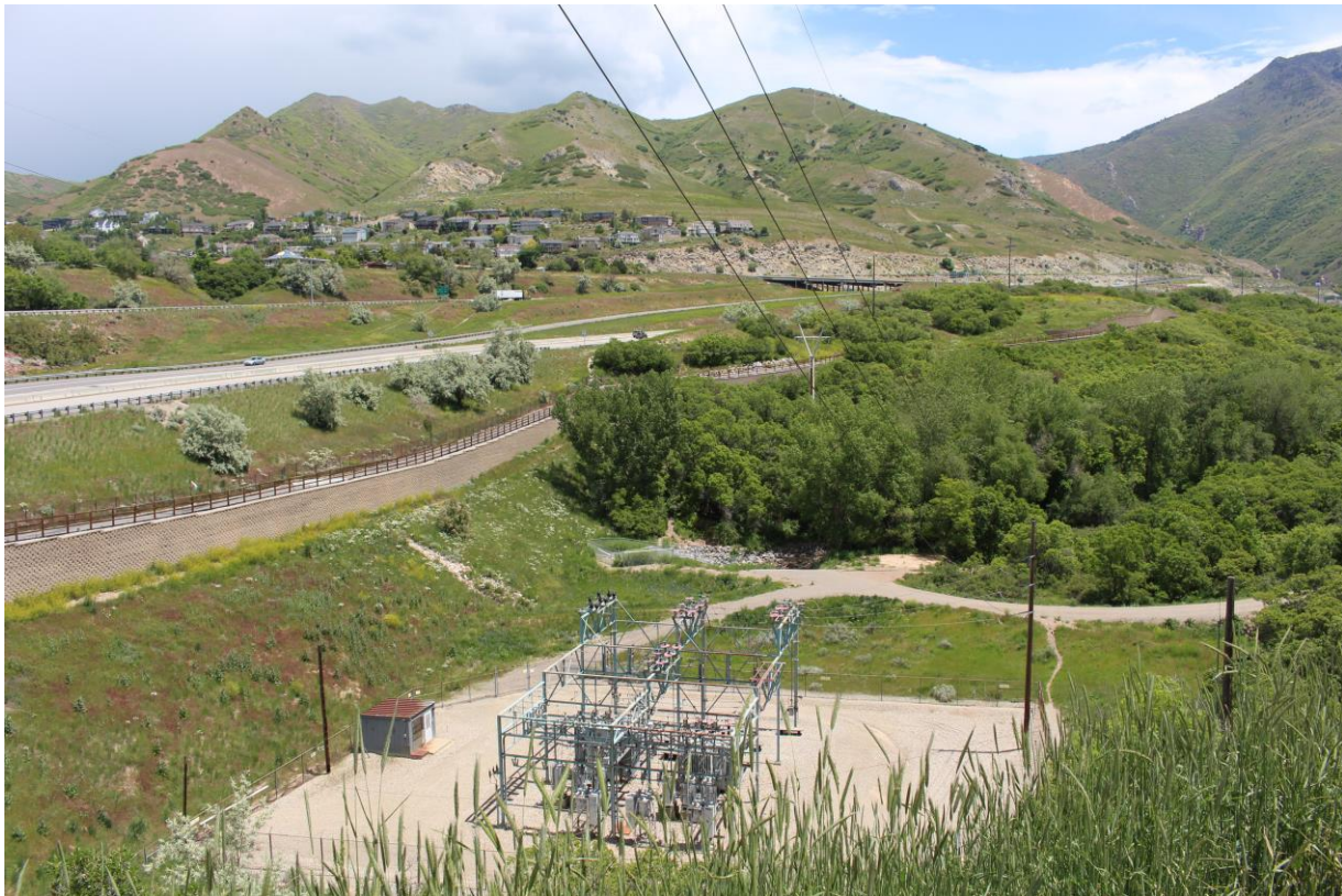
Fig. 82. View to the east overlooking the "West Off-Leash Dog Area" and Parley's Creek Corridor Trail which follows along the northern perimeter of the park. Photograph taken from the Parley's Creek Corridor Trail western extent of the park (JoEllen Grandy, 5/27/16).
