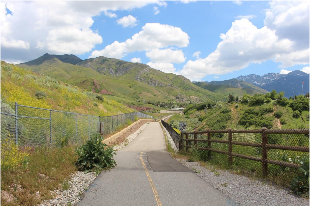
Fig. 62. View to the east of Parley’s Creek Corridor Trail located north of the “East Off-Leash Dog Area”. Note the block retaining wall and chain link fencing (JoEllen Grandy, 5/27/16).
