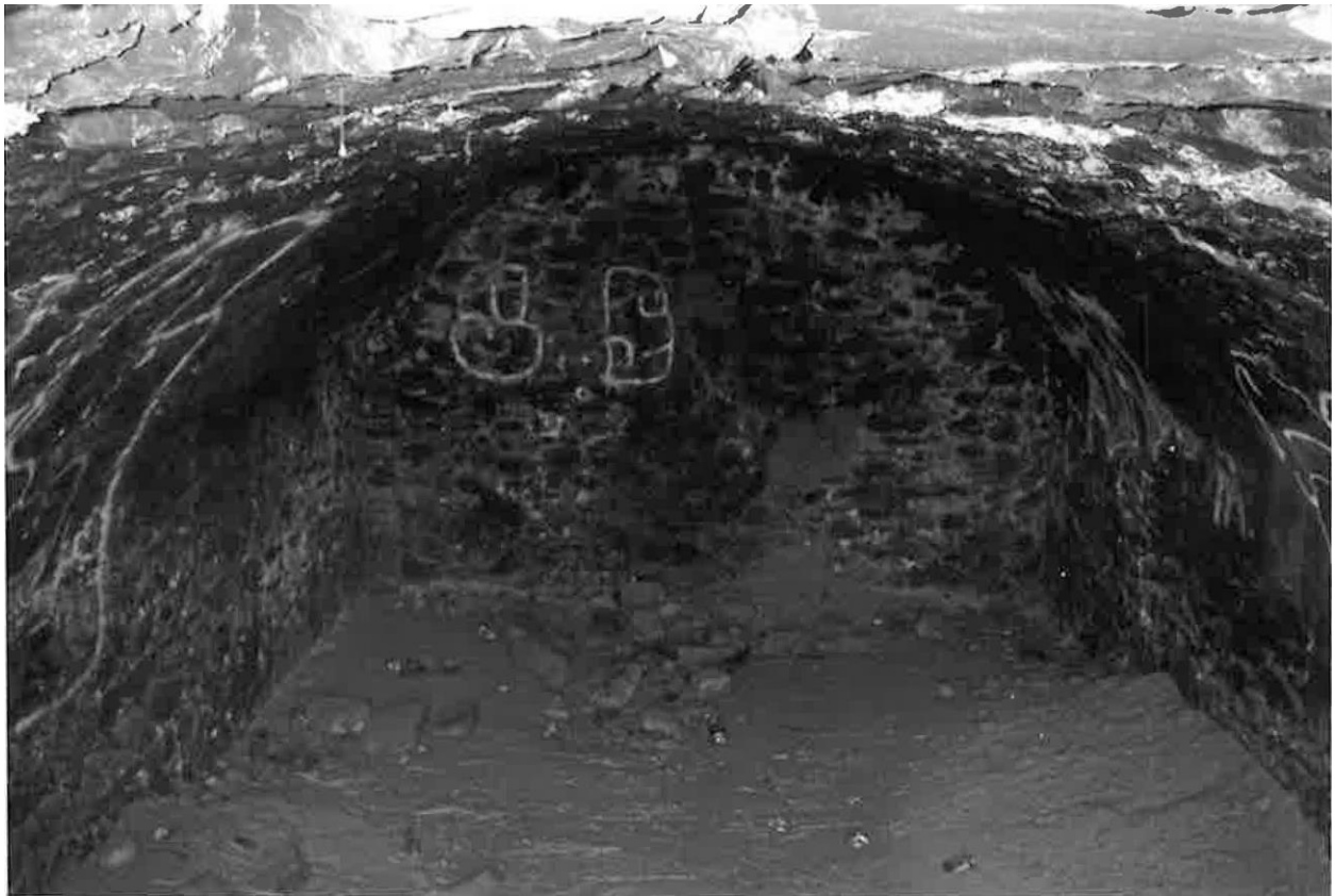
Fig. 122. Close-up view to the north inside the wine cellar. Photograph taken in 2007 (Simms, Dudler).
