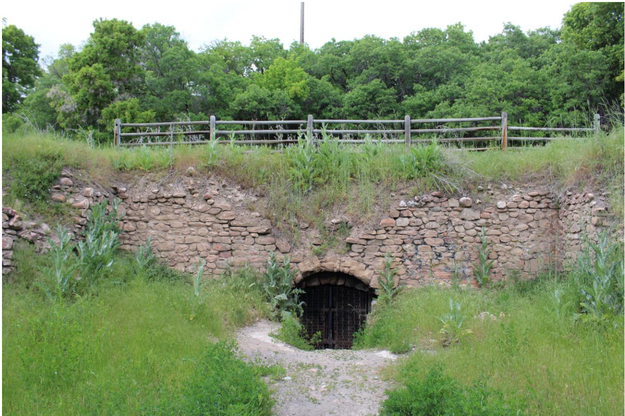
Fig. 74. Close-up view to the north of remnants of Dudler's Wine Cellar located on the northside of Parley's Creek Corridor Trail, immediately north of the large boulder monument. Note the gated entrance into the cellar (JoEllen Grandy, 5/27/16).
