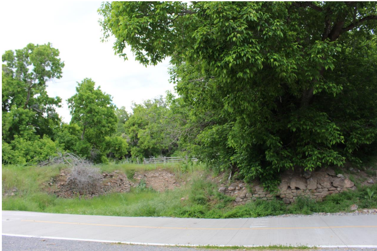
Fig. 71. View to the northwest of remnants of the Dudler's Inn (stone wall to the right near the trail) and Wine Cellar (to the rear left) located on the northside of Parley's Creek Corridor Trail, immediately north of the large boulder monument (JoEllen Grandy, 5/27/16).
