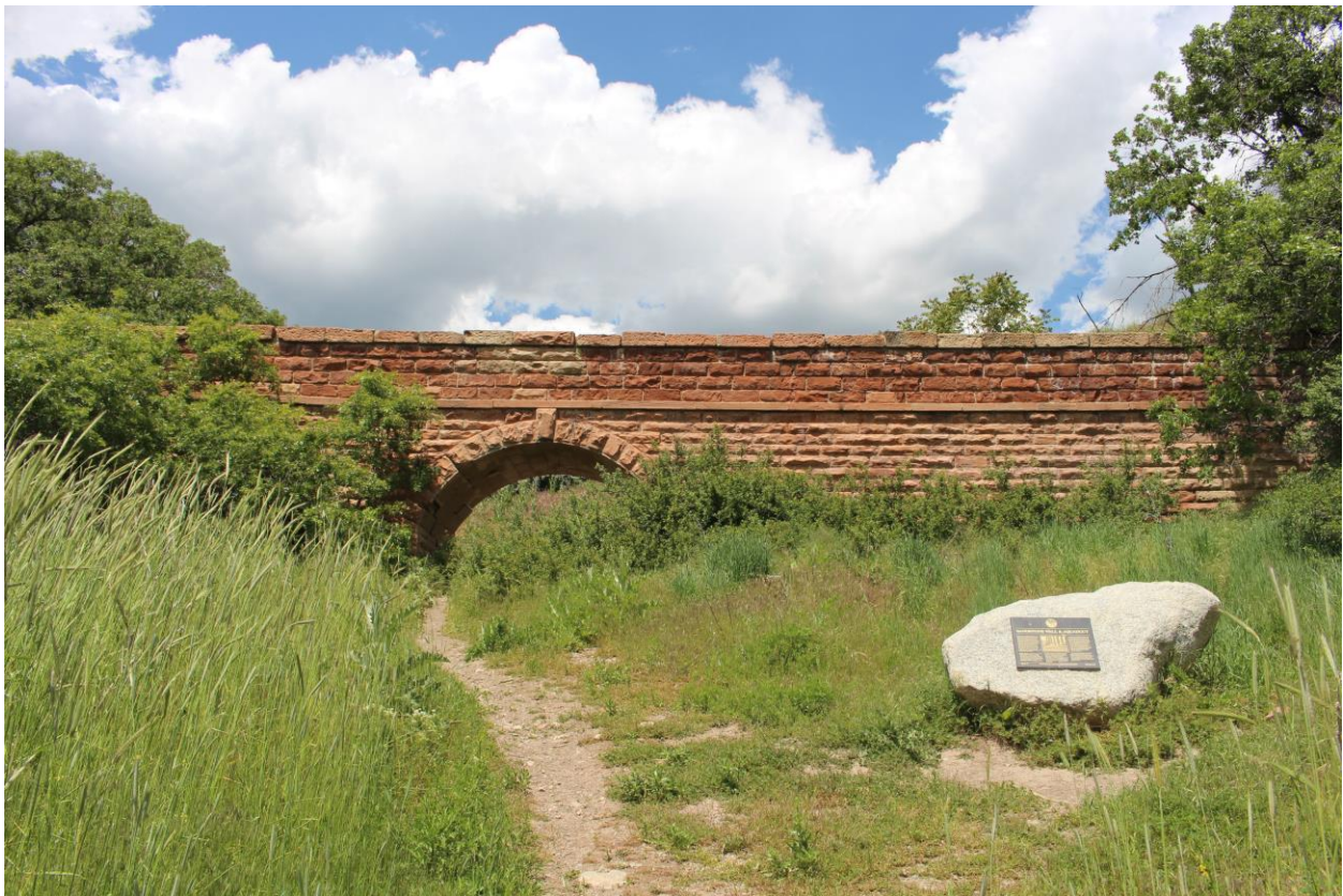
Fig. 78. Close-up view to the north of the historic sandstone wall and aqueduct built circa 1891. Note the large boulder monument to the right (JoEllen Grandy, 5/27/16).
