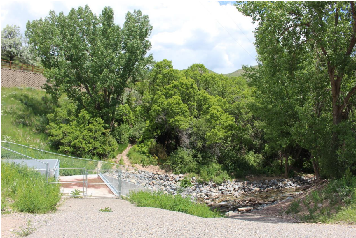
Fig. 32. View to the northeast of Parley's Creek as it is channeled into a culvert, slightly northeast of Rocky Mountain Power's Parley's Substation located in the far west end of the park (JoEllen Grandy, 5/27/16).
