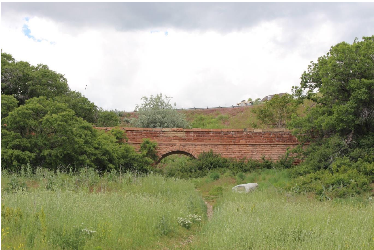
Fig. 111. Approaching view to the north of the historic sandstone wall and aqueduct built circa 1891 located on the northside of Parley's Creek Corridor Trail, slightly west from Dudler's Inn and Wine Cellar remnants. Photograph taken in 2016 (JoEllen Grandy, 5/27/16).
