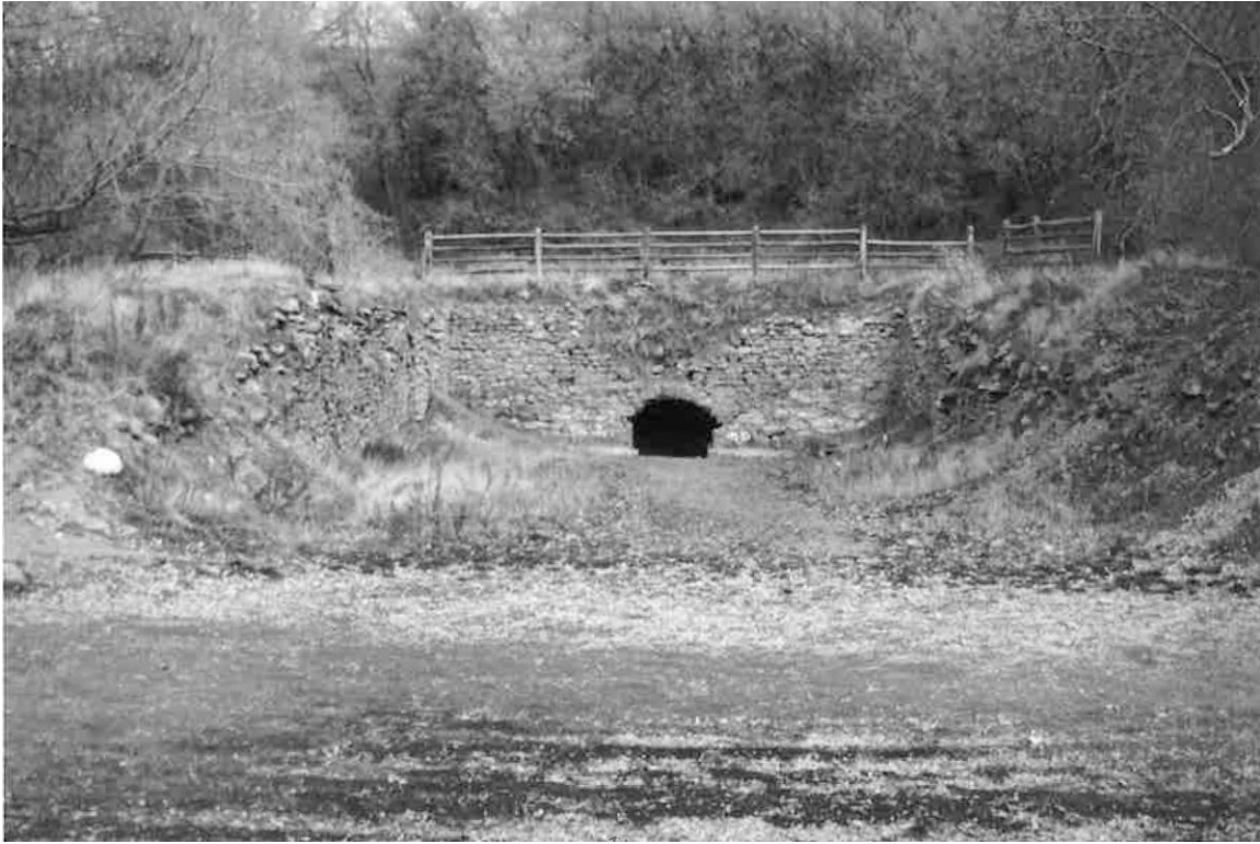
Fig. 120. View to the north of remnants from Dudler's Wine Cellar. Photograph taken in 2007. Compare with fig. 73 in 2016 (Simms, Dudler).
