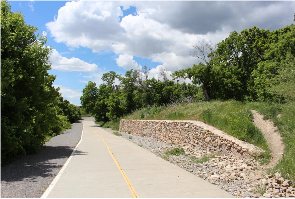
Fig. 66. View to the west of a stone retaining wall, located slightly east from the remnants of Dudler’s Inn and Wine Cellar, northeast of the “Central Off-Leash Dog Area” and northwest of the “East Off-leash Dog Area and The Golden Pass Road and Tollhouse marker, on the north side of Parley’s Creek Corridor Trail (JoEllen Grandy, 5/27/16).
