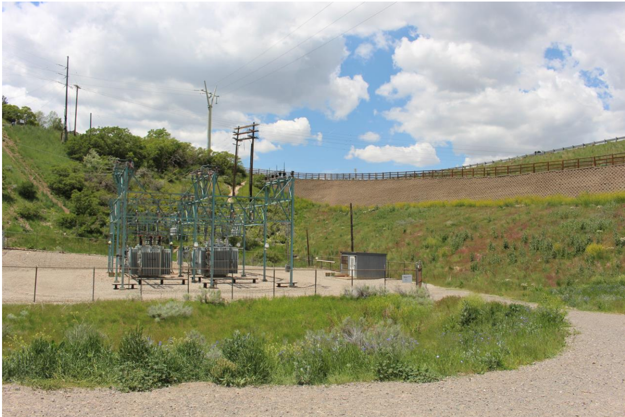
Fig. 31. View to the northwest of the Rocky Mountain Power’s Parley’s Substation located in the far west end of the park. Note in the upper left corner along the rim of the hollow, Parley’s Creek Corridor Trail (JoEllen Grandy, 5/27/16).
