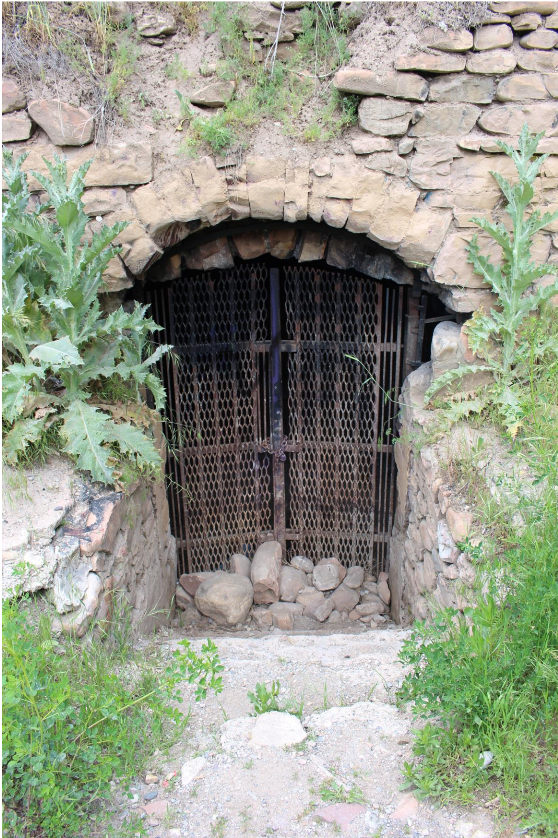
Fig. 75. Close-up view to the north of the entrance into the wine cellar (JoEllen Grandy, 5/27/16).
