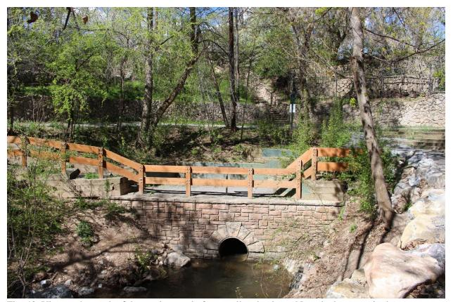
Fig. 40. View to the north of the sandstone platform wall and culvert. Note the keystone in the masonry arch outlining the culvert (JoEllen Grandy, 4/11/16).
