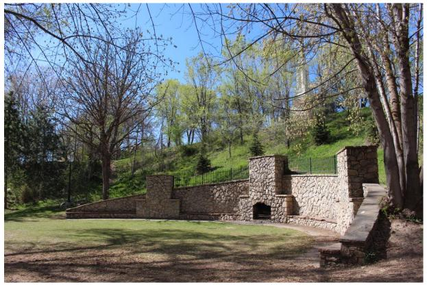
Fig. 100. View to the northwest of the crescent-shaped stone retaining wall with originally three fireplaces. Note two of the three have been sealed (JoEllen Grandy, 4/11/16).
