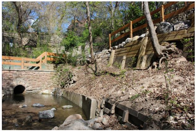
Fig. 41. View to the northeast of the crib walls and reinforced concrete, boulder and timber walls located along the eastern edge of the creek near the culvert (JoEllen Grandy, 4/11/16).
