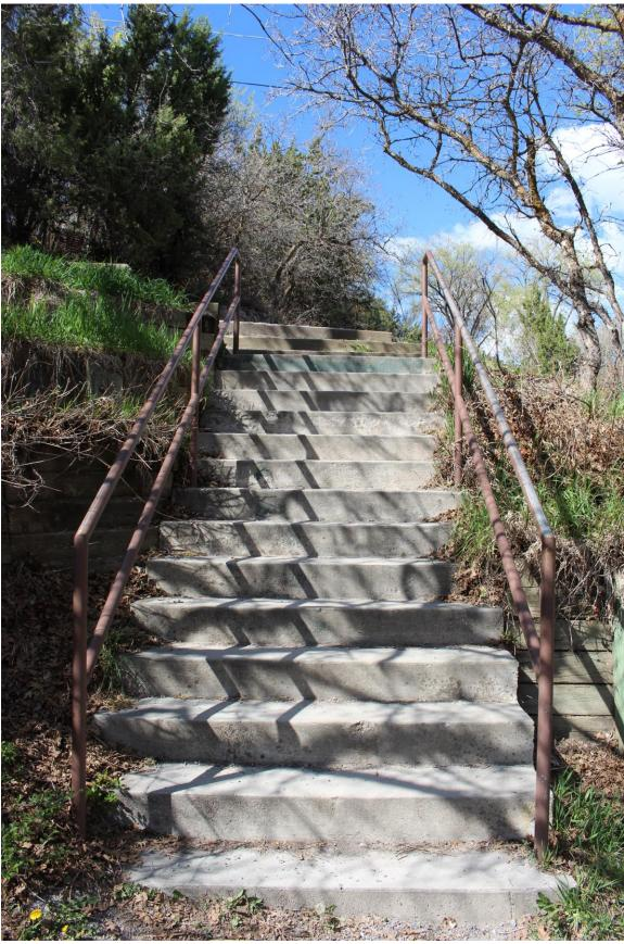
Fig. 71. View to the northeast looking back toward the concrete staircase connecting access to the west perimeter trail. Note the timber retaining walls each side of the stairs (JoEllen Grandy, 4/11/16).
