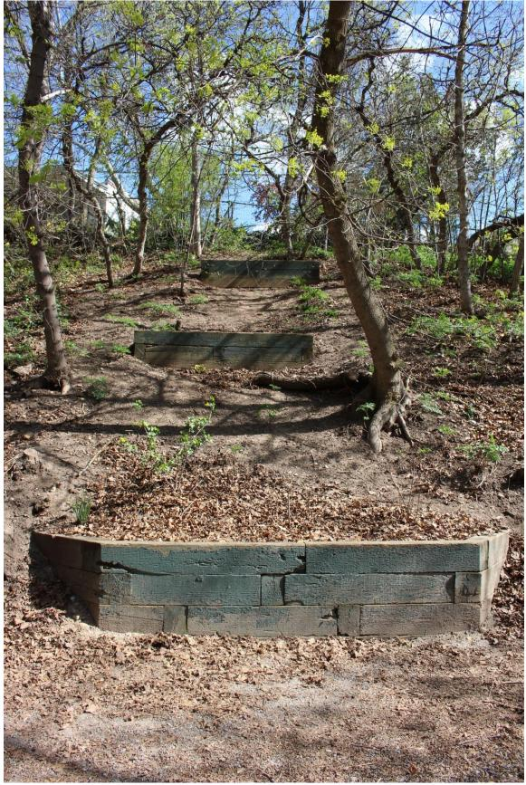
Fig. 87. View of a three terraced timber retaining wall located directly southeast of the bridge to help slow potential erosion (JoEllen Grandy, 4/11/16).
