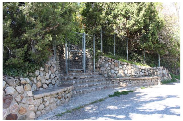
Fig. 67. Northeast bound view of the cobblestone flight of staircase to Diestel Road. Note the built-in cobblestone seating into the retaining wall either side of the stairs (JoEllen Grandy, 4/11/16).
