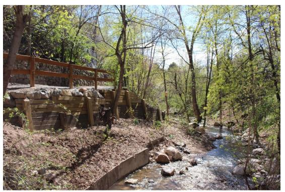
Fig. 39. View to the south of a portion of the crib and reinforced concrete wall located along the eastern edge of the creek near the culvert in 2016. Note the relocation of the eastern perimeter trail following the perimeter of the retaining wall in the top left corner and additional timber retaining walls and the removal of the chain link fencing and separation from the creek below (JoEllen Grandy, 4/11/16).
