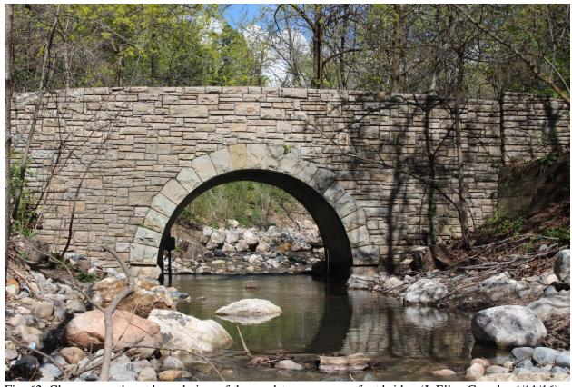
Fig. 62. Close-up northeast bound view of the sandstone masonry foot bridge (JoEllen Grandy, 4/11/16).
