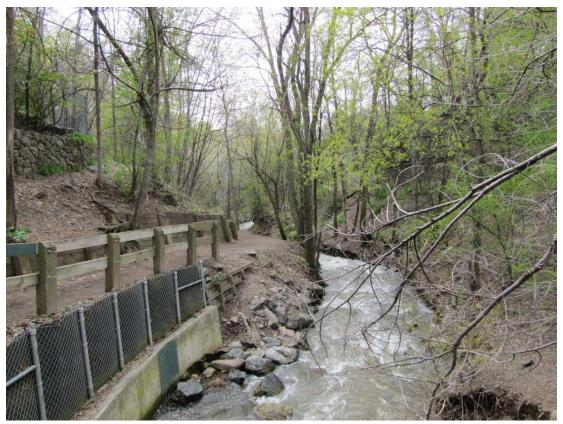
Fig. 38. Undated view to the south of a portion of the crib and reinforced concrete wall located along the eastern edge of the creek near the culvert. Note the location of the eastern perimeter trail in relation to the creek, and retaining wall in the top left corner (Parks).
