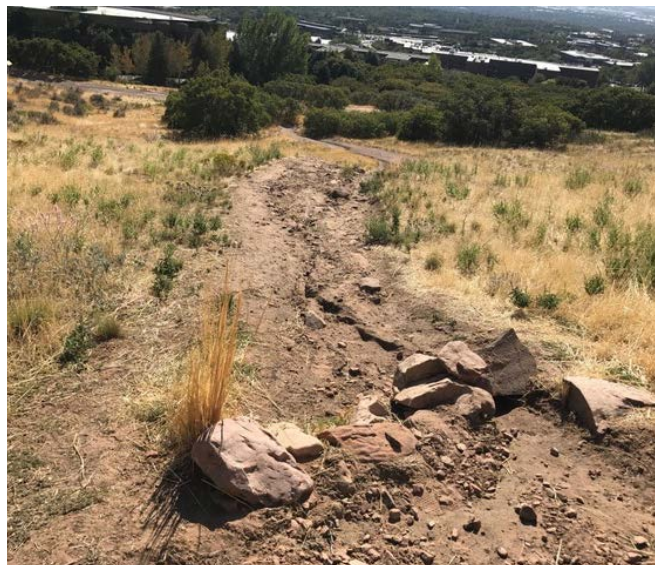
Fall line trails, such as the one, above are prone to erosion and rutting.
