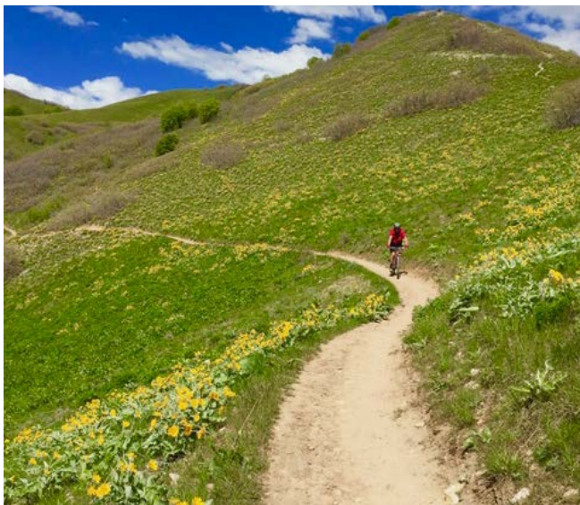
Trails that follow existing contours are less prone to erosion and are accessible by a wider range of trail users
