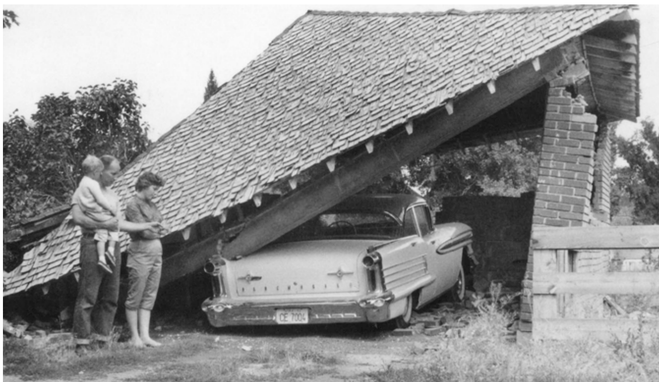
Figure 9. URM pier failure. Photo: Ariel Benson
