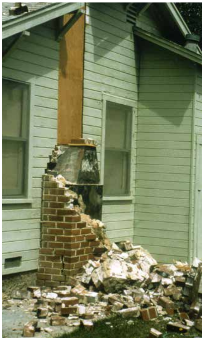
Figure 12. Chimney collapse.
