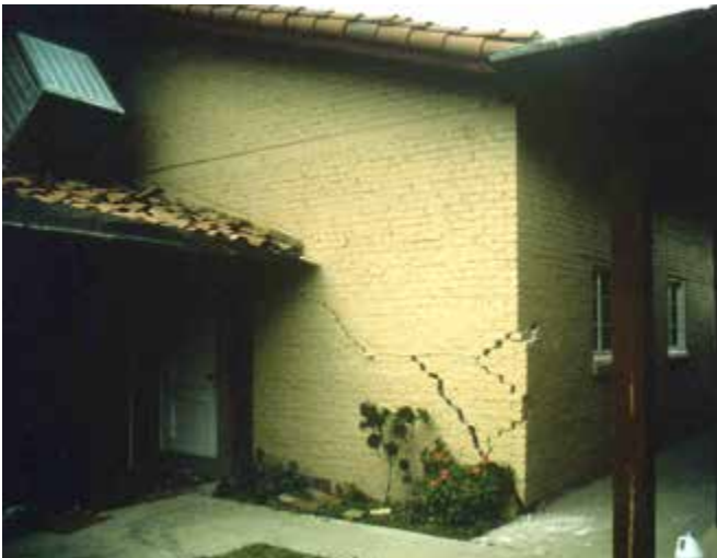
Figure 7. Earthquake damage to an URM wall and displacement of mechanical equipment on roof.
