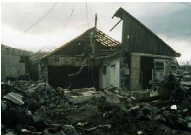
Figure 3. URM structure collapse.
