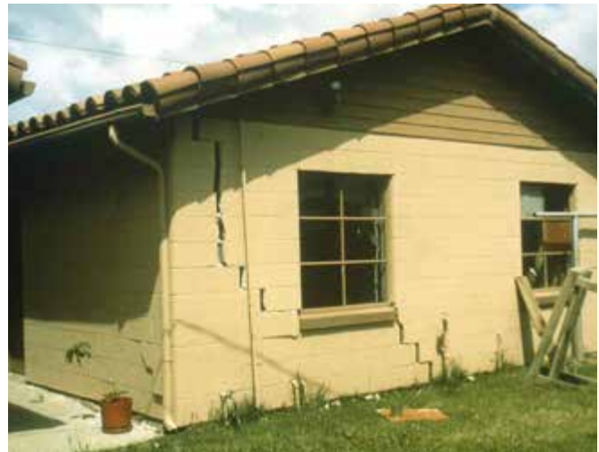
Figure 8. URM wall failure from an earthquake.
