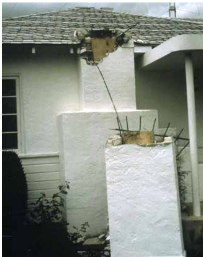
Figure 11. Chimney failure due to inadequate reinforcement.
