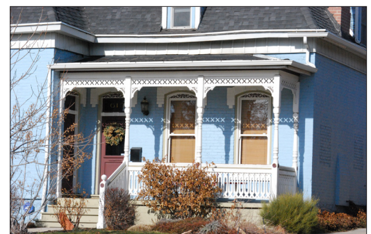
The detailing of a porch, whether entablature and columns or this jigsaw ornamentation with intricate balustrade, should be preserved.
