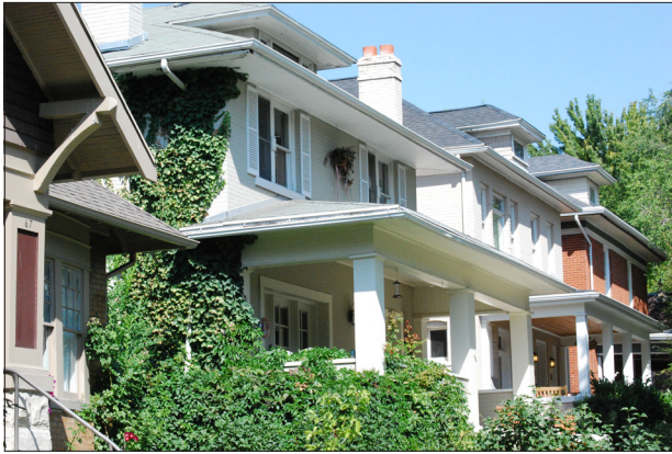
Square columns in various designs create detailed variety and a visual richness in this complementary sequence of full-width porches.
