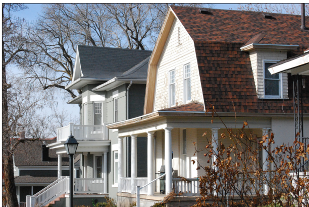
Porch design is usually a notable part of the architectural style and composition, articulating building orientation and scale, while emphasizing intricate detailing and craftsmanship.
