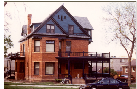
Avenues home after rehabilitation, Salt Lake City
