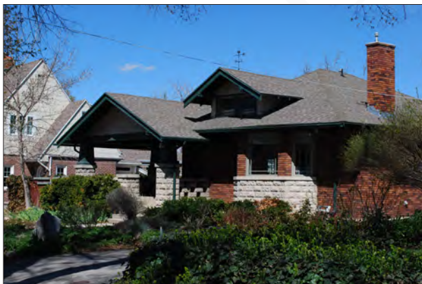
The architectural character of the building incorporates a variety of traditional design characteristics such as external porch, deep eaves, natural ventilation and solid masonry construction, ensuring efficient energy management and conservation.
