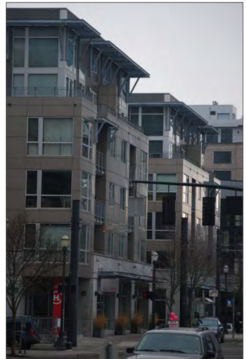
Symmetrical massing, emphasized by recessed vertical balcony bays, setting back top floors, and varied fenestration create both a distinct vertical proportion and sense of human scale.
