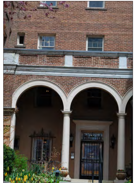
The collonade establishes the importance of the entrance court and the entrance.
