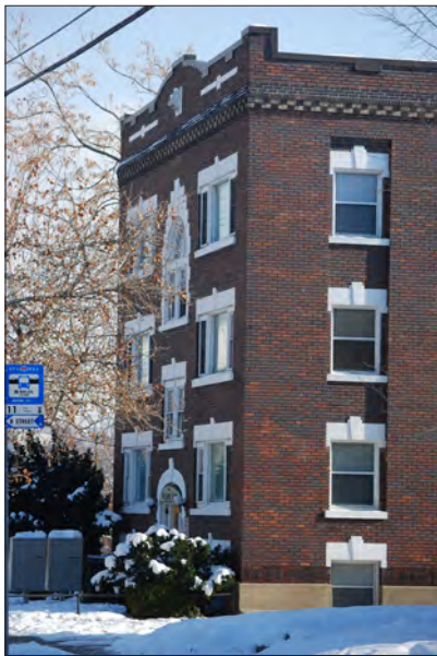
Wilshire Arms Apartments
