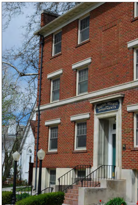
Federal Heights Apartments
