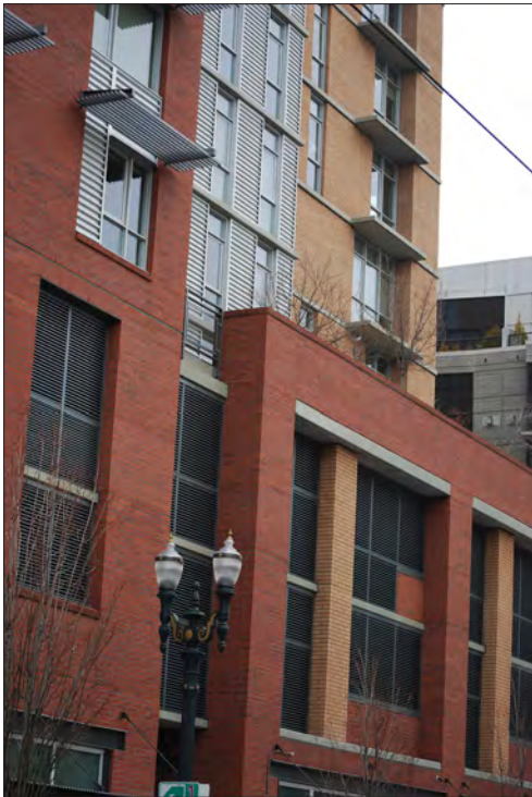
Brickwork employed as a decorative expression of architectural style, and effectively conveying a sense of human scale within a taller building.
