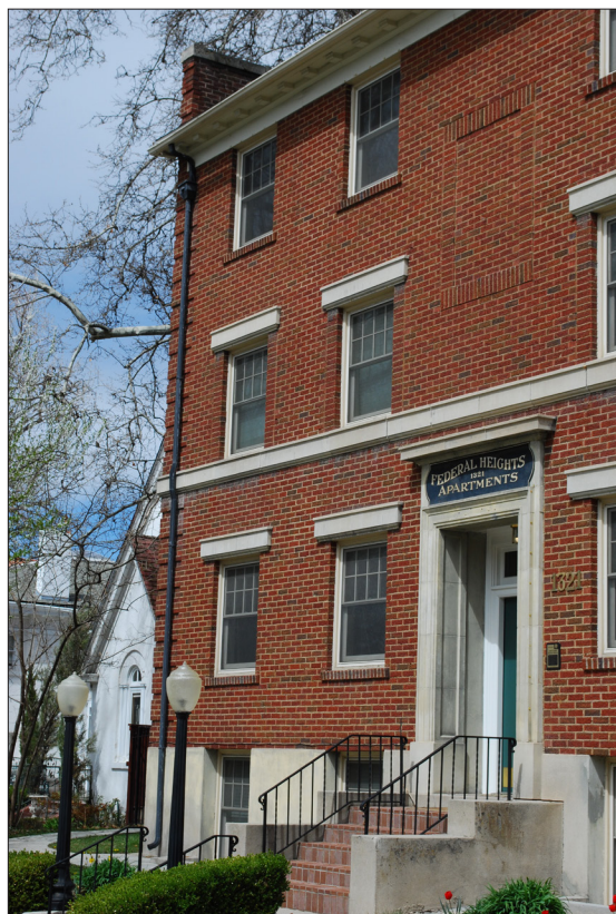
Federal Heights Apartments
