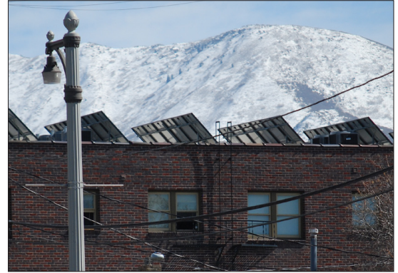
Building utility locations can have unanticipated consequences.
