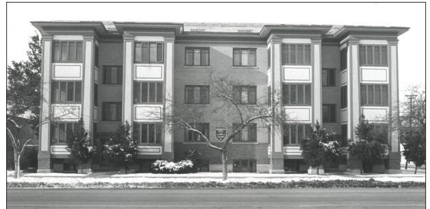
Browning Apartments, c. 1916, Ogden, Weber County. Constructed for Ogden businessman George E. Browning, this horizontal block shows the influence of the Prairie School style in the use of casement windows and wood banding.
