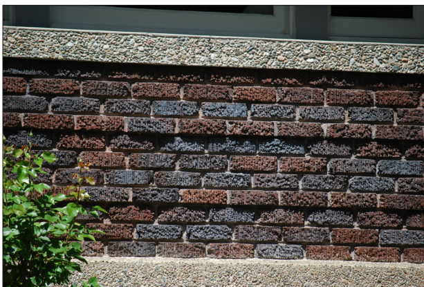
A decorative choice and use of materials, detailing and textures combines thermal mass with low maintenance.
