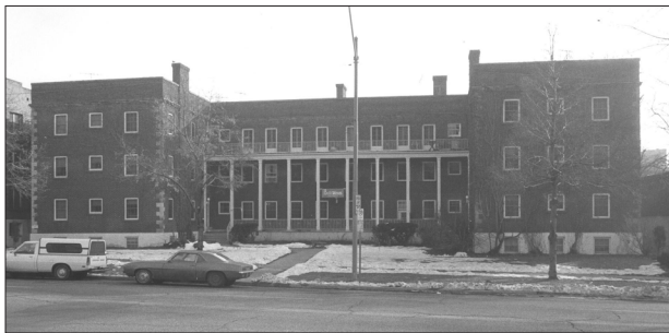
Bell Wines Apartments, 1927, Slack Winburn, architect, Salt Lake City, Salt Lake County. This "H"-type apartment block is preceded by an unusually shallow forecourt. A tall portico supported by square columns spans the width of the court. The wings of the building are emphasized by stone quoins and a molded cornice.
