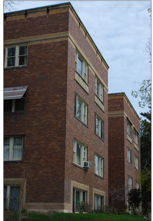
Symmetrical projecting wings of the primary street facade enclose a central recessed entrance court.
