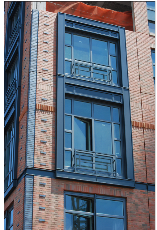
New construction using dark metal framed vertical window bays set within a complimentary and contemporary decorative brickwork facade.
