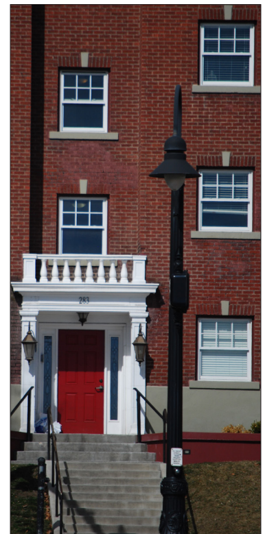
From street light to principal entrance.
