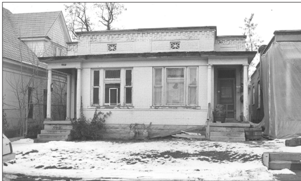
Double house, c. 1905, Salt Lake City, Salt Lake County. This single-story example of the double house has side entries with narrow porches supported by Tuscan columns.
