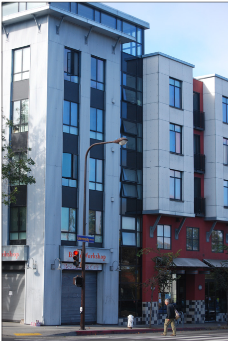
Articulation of the street facade, varying the planes, materials and facade proportions, help to integrate the commercial street frontage and create a sense of human scale.
