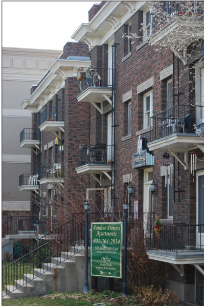
Symmetrical massing and composition, balconies and fenestration pattern combine to integrate with the street.
