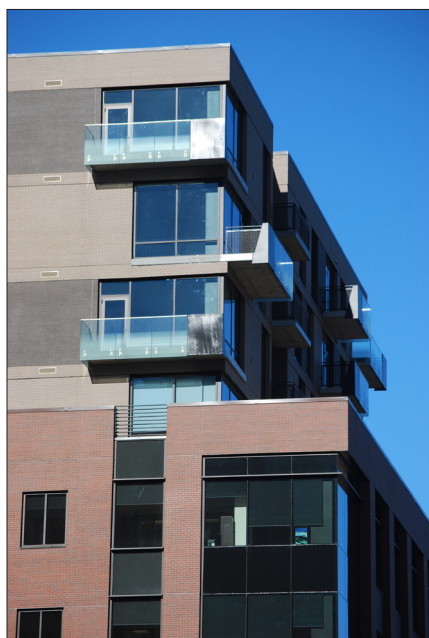
Alternating pattern of windows and balconies, with well-considered detailing and materials, articulate and reduce the apparent scale of the building.
