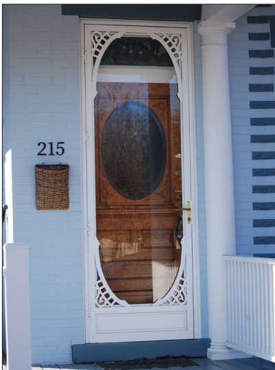
An exterior storm door revealing the detailing of the original behind.
