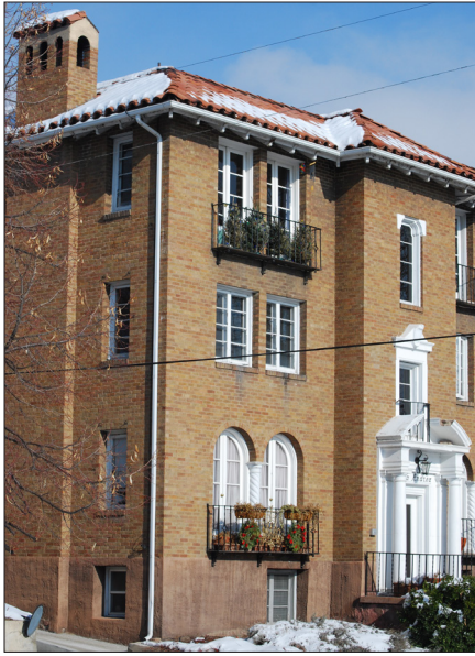
Projecting central entrance and bay, full height chimney and vertically proportioned window sequence, create strong verticality.
