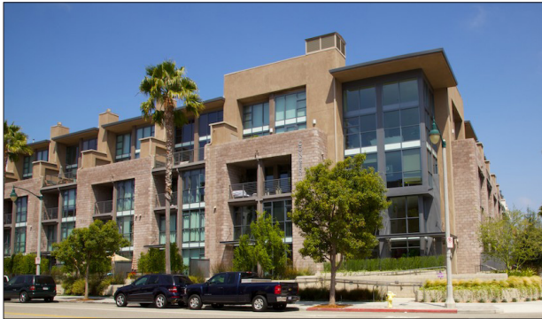
Stepping back the top floor combines with facade articulation and corner design focus to reduce perceived height and scale.
