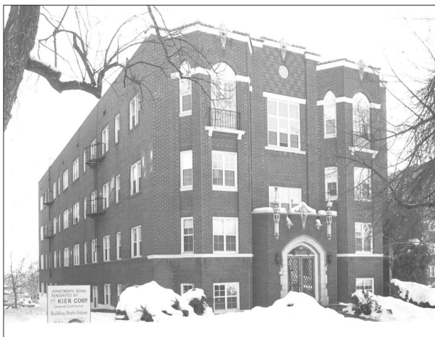
Kier Corp. Apartments, c. 1932, Salt Lake City, Salt Lake County. A projecting central entry complete with terra-cotta surround and decorative finials is flanked by two projecting bays that articulate the facade and distinguish this apartment building from its neighbors.
