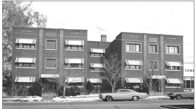
Rose Apartments, 1923-24, Ogden, Weber County. This is a brick masonry “C”-shaped apartment building containing entries in the wings.
