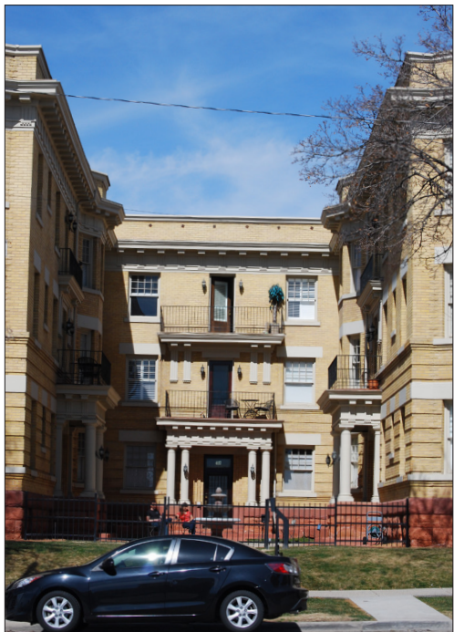
A Classical celebration of the central street-facing court in the detail of doorways, balconies, brickwork and stone detailing, creating an intimate sense of human scale.
