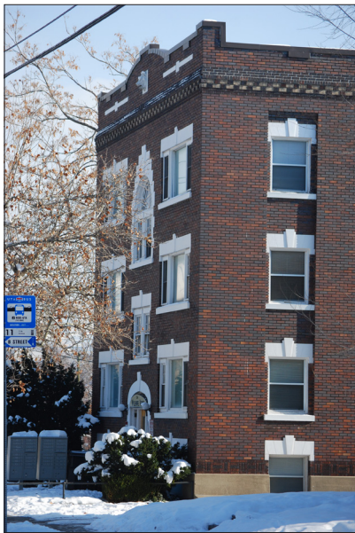
Wilshire Arms Apartments
