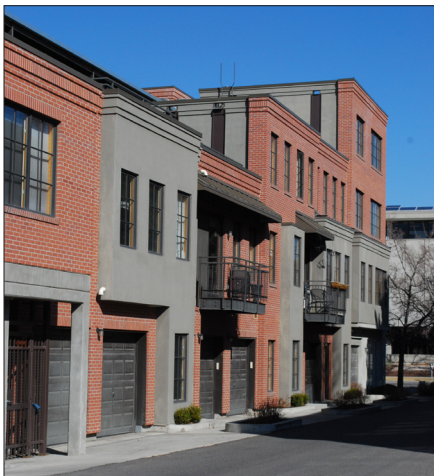
Stepping down massing towards the rear of the building.
