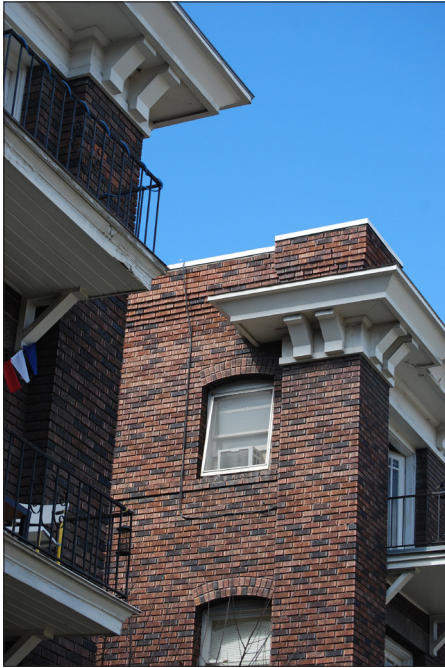
Cornice and balcony profiles and decorative brackets tie together the design detail of railings, windows and brickwork.
