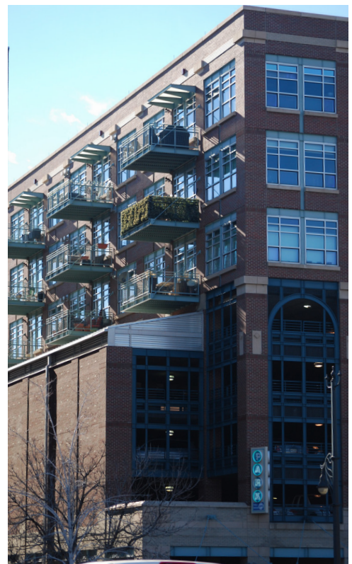
The window frame pattern and profiles effectively used to embellish facades and screen parking decks.
