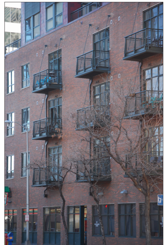
Fenestration pattern, accentuated by projecting balconies, helps to define the rhythm and proportion of the street facade.
