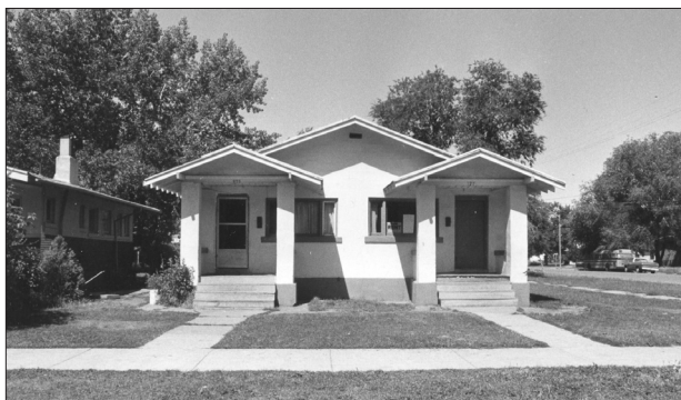
Double house, c. 1915, Salt Lake City, Salt Lake County. Separate gabled entries project from this double house, built in the style of a California bungalow with low pitched roofs, exposed rafters, and stucco over wood frame construction.
