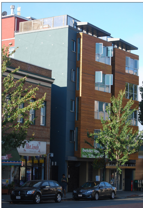
Recessed garage access from the street with minimal interruption of the street frontage.
