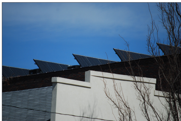
Solar collector panels are becoming increasingly affordable and are being developed in a variety of forms and scales, as with this installation on a traditional apartment building.
