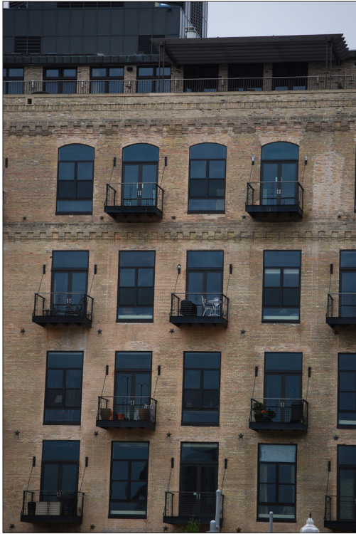
The recent addition of individual alternating projecting balconies has been used effectively to redefine and articulate the character and interest of the warehouse facade.
