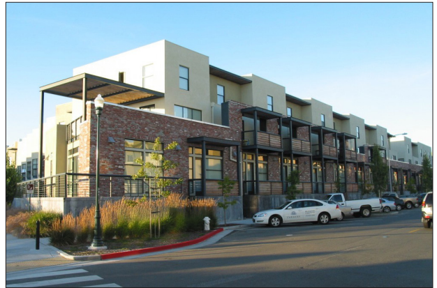
A lower facade of quality materials supports a strongly articulated street facade with a distinct vertical proportion and rhythm in this horizontal building.
