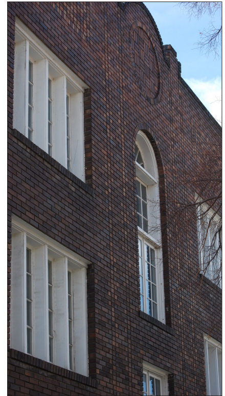
Stone window reveals and mullion subdivision contrast with the dark brickwork of the facade wall.
