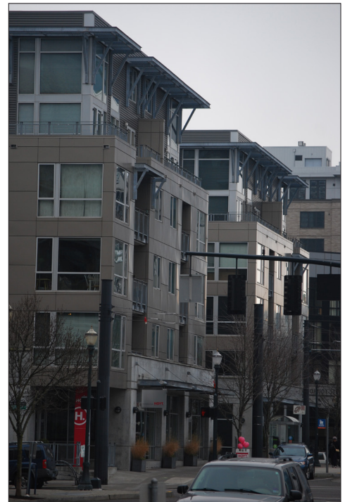
Symmetrical massing, emphasized by recessed vertical balcony bays, setting back top floors, and varied fenestration create both a distinct vertical proportion and sense of human scale.
