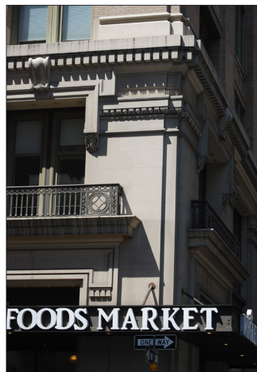
Signs and lettering design can reflect and also enhance the building.
