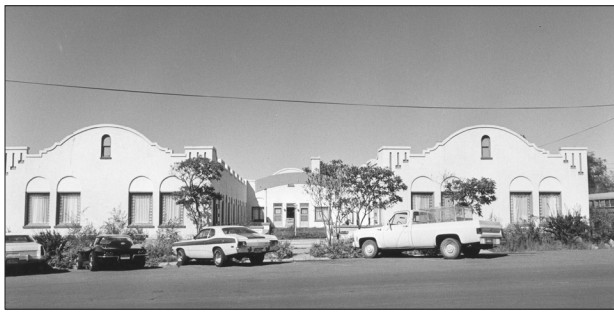
Apartment court, c. 1920, Price, Carbon County. A one-story “U” court of stuccoed masonry, this apartment building shows the influence of the Mission style.
