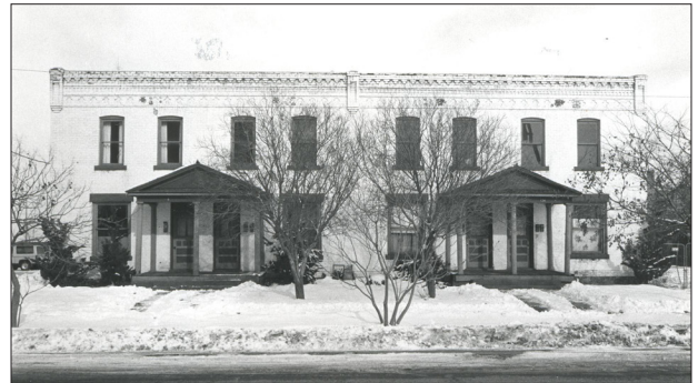
Four-unit block, c. 1900, Ogden, Weber County. This example of the four-unit block contains separate entries for each apartment and a unified corbeled brick cornice and parapet.
