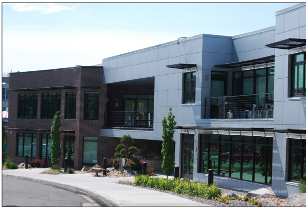
A contrast in facade design and materials, and the modeling of the facade can help to break down the lateral scale, while enhancing the visual interest and presence of the building.
