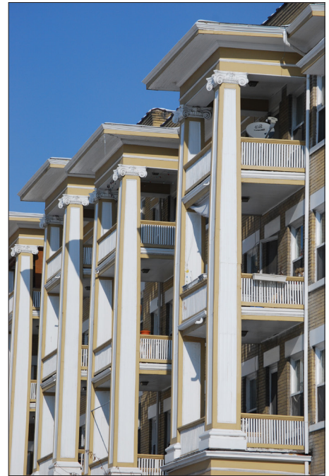
Slender columns support an equally slender sequence of terraced balconies and create a vibrant vertical emphasis and proportion across an extensive historic apartment complex.
