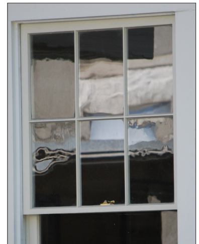
The reflective ripple characteristics of early glass can be appreciated when compared to the regular surface of more recent replacement glass.
