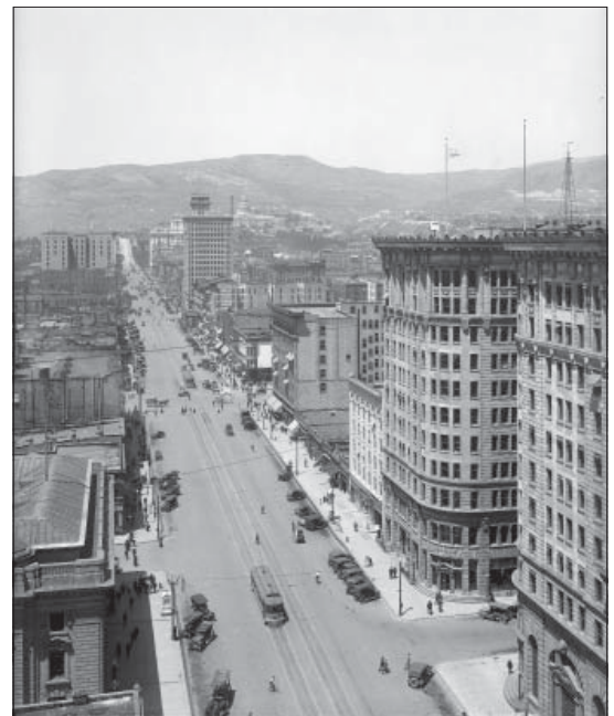
Skyscrapers, like the 11-story Boston Building (1909), at Exchange Place and Main Street, became more common with the development of a lucrative mining economy.
