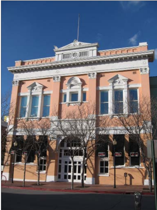
Identify, retain and preserve buildings of character, 122 West Pierpont Avenue.
