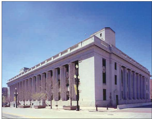
The Federal Building and former Post Office at 350 S. Main Street (1906) is an example of an enframed block designed in the Neoclassical style. The building is distinguished by its long row of engaged Doric columns on each facade.
