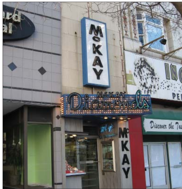
The McKay Jewelry Company at 157 S. Main Street (ca. 1950) features a restrained upper facade and original aluminum and glass storefront.
