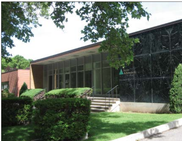
The building at 641-645 E. South Temple Street (1957) displays black marble panels and a sleek exterior.
