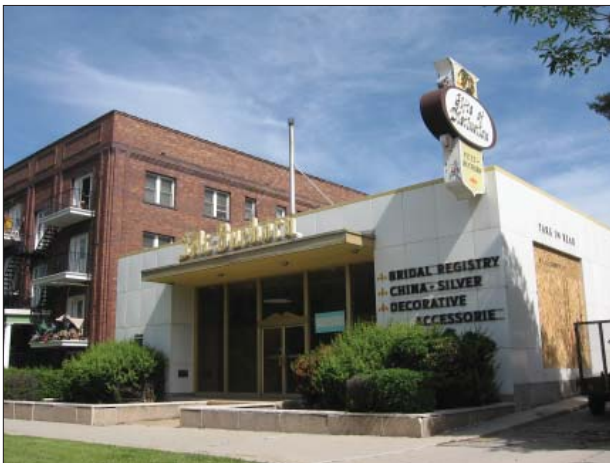
An enframed window wall plan is the Felt-Buchhorn Building at 445 E. South Temple Street (1959). It displays a continuous surround of porcelain steel panels which frame the display windows and entrance.
