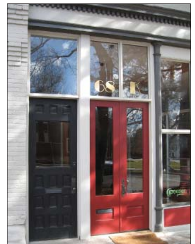
Salt Lake City's commercial buildings have a variety of doors and entrances.
