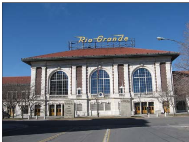
The State Historic Preservation Office is located in the Denver & Rio Grande Railroad Station at 300 South Rio Grande Street.
