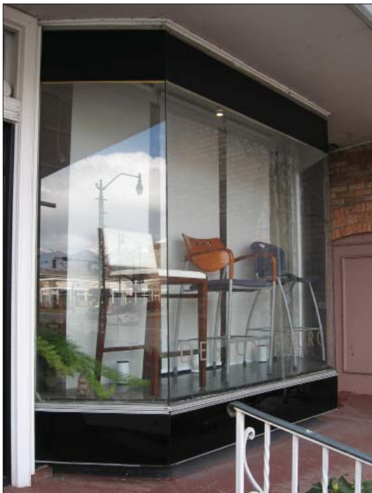
The Carrara glass is a distinctive characteristic of the storefront at 432-434 E. South Temple Street.
