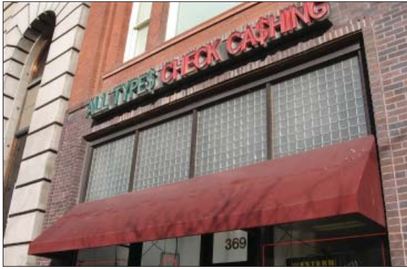
The distinctive Luxfer glass transom on the New Grand Hotel at 369-379 S. Main Street is intact and not concealed by the awning.
