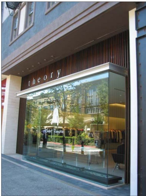
This contemporary interpretation of a traditional storefront features a display window that is predominantly transparent glass.
