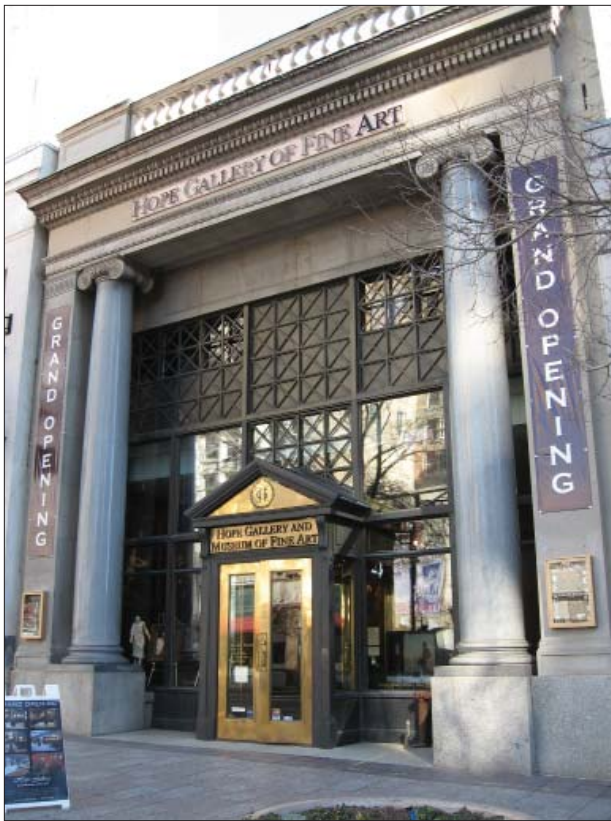
The Tracy Loan Trust Company (1916) was constructed at 151 S. Main Street. This vault design features a large central bay with a pedimented entrance flanked by Ionic columns. In addition to the entrance, the central bay is composed of a large window wall.
