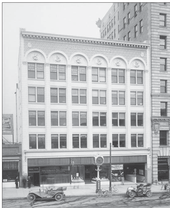
The Felt Building (1910) at 339 S. Main Street displays early use of terra-cotta as a decorative element.
