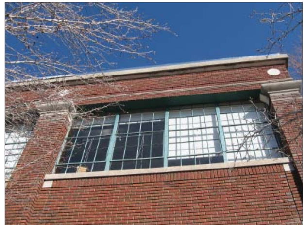
Steel frame windows are characteristic of many historic buildings of the 20th century.
