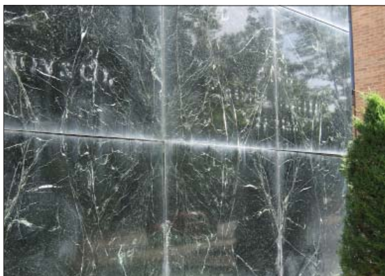
Marble paneled veneer on the main facade at 641-645 E. South Temple Street.
