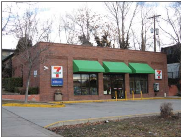
This simplified version of a one-part commercial block, while a compatible design could have been improved by stepping it forward to the street frontage. The rear of the building would have been a better location for the surface parking.
