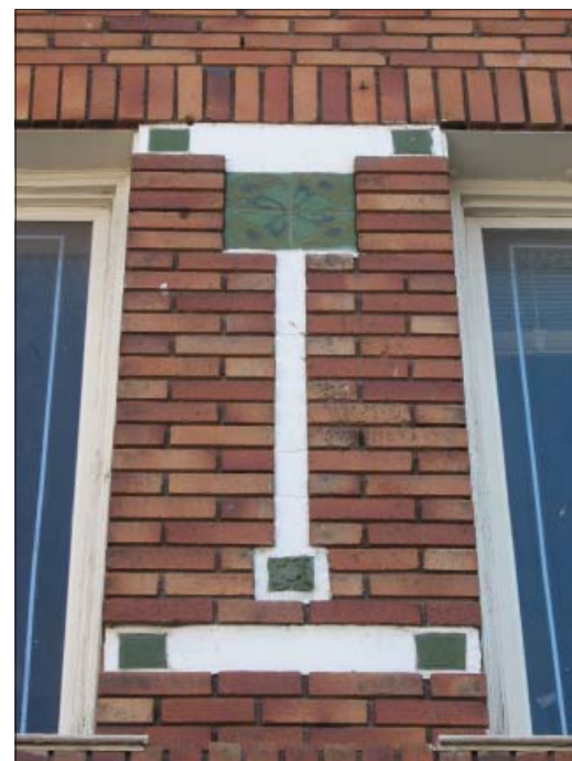
Architectural details help to define the distinctive visual character of this historic building at 145 S. State Street.
