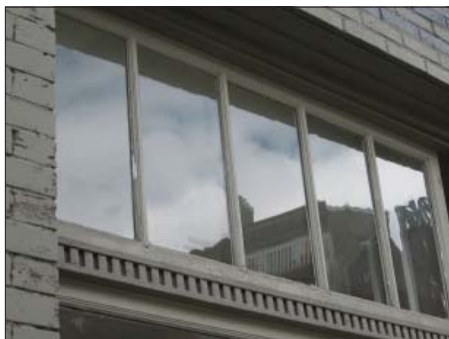
Original transoms contribute to the character of this historic storefront at 271 N. Center Street.
