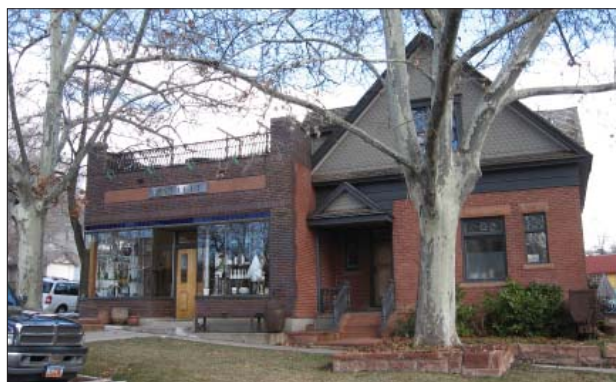
This building at 82 North 'Q' Street (1898) features an original storefront in the commercial section.
