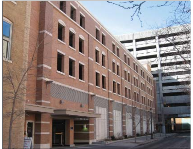
Site multi-story parking lots in the downtown area at interior areas of the block; design them to screen vehicles as much as possible, such as this garage in the 100 block of State Street.
