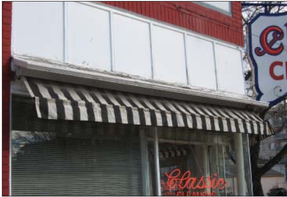
The awning fits within the window opening at 501 East 300 South.
