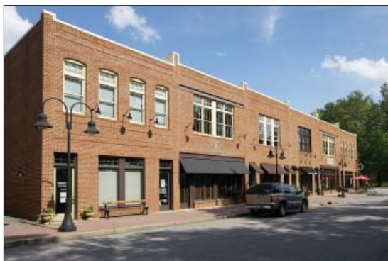
Smaller building “modules” can be expressed within a single building using variations in window patterns and cornice detailing.
