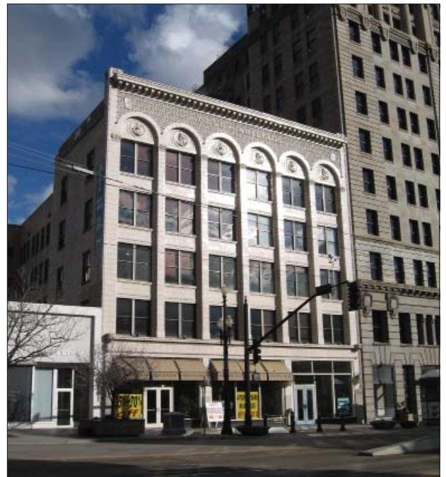
The Felt Building at 335-339 S. Main Street (1909) has a separate storefront zone and unified upper facade. The building is distinguished by its glazed terra-cotta and arched panels below the cornice.
