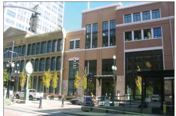
A step back provides a transition between the historic ZCMI storefront and the infill construction.
