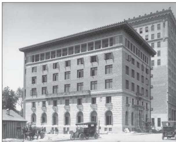
The Commercial Club Building (1908) borrows its architectural detailing and overall style from the Second Renaissance Revival style.
