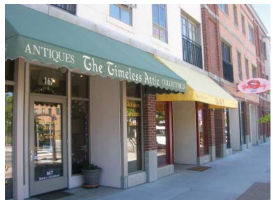
Awnings add color and enliven storefronts while enhancing the character of the street scene.
