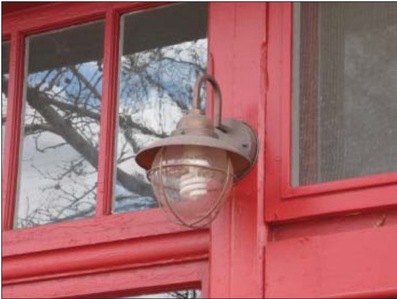
Good lighting choices for historic buildings are simple and unobtrusive, such as this example at 361 N. Main Street.
