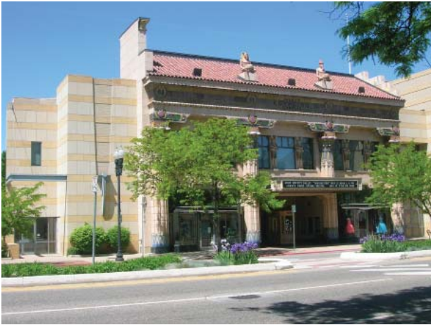
Variations in setback and materials can provide a visual distinction between the historic building and its addition.
