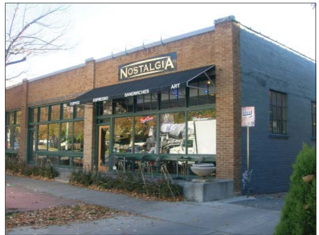
Most historic commercial buildings were designed with flat or gently sloping roofs.
