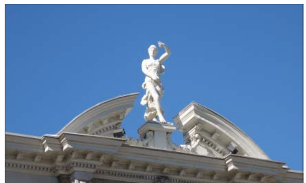
Decorative elements such as this statue at the Promised Valley Theatre are part of a building's unique roof profile.
