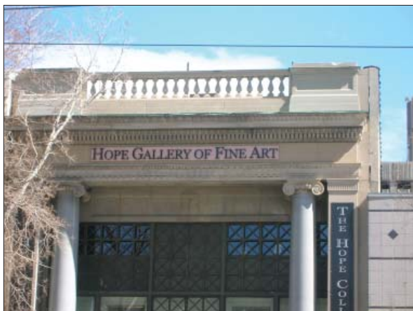
Cornices and balustrade add classical detailing to the street facade at 151 S. Main Street.
