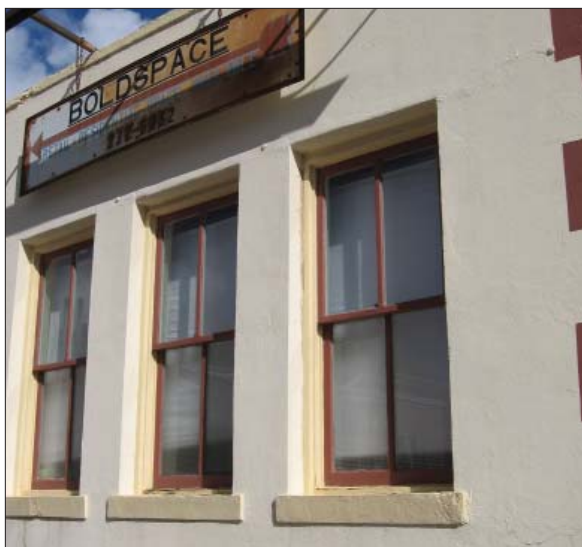
The number and position of glass panes in a window are important character-defining features of a building.
