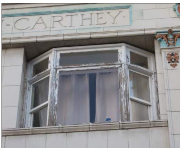
Regular maintenance is essential and will markedly improve the longevity of a historic window.
