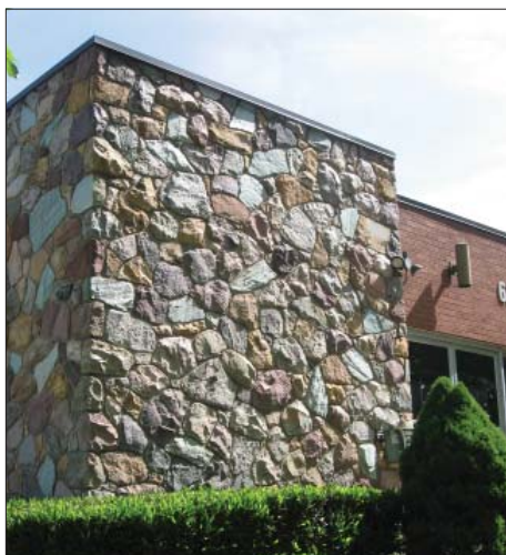
This stone veneer corner bay is at 633 E. South Temple Street.
