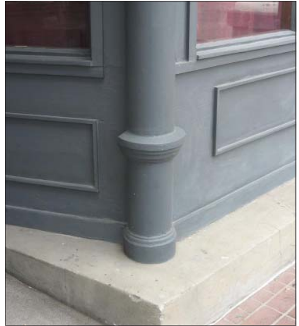
Decorative metal detailing is a significant characteristic of the street facade.
