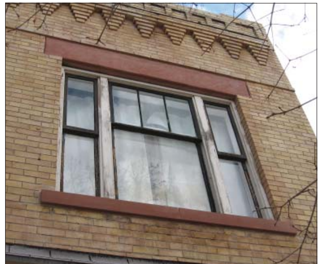
The wood framing distinguishes this historic window design, profile and detailing in an upper story window treatment.
