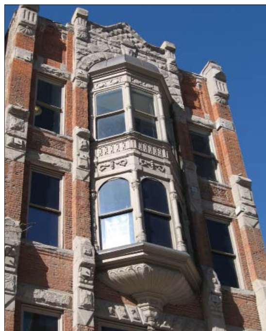
The decorative combination of contrasting masonry materials, color and texture is used to full architectural effect at 328 S. Main Street.
