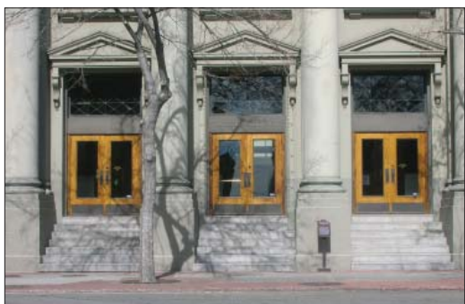
These three center bays are framed by four freestanding Ionic columns. Salt Lake Stock and Mining Exchange, 39 Exchange Place.
