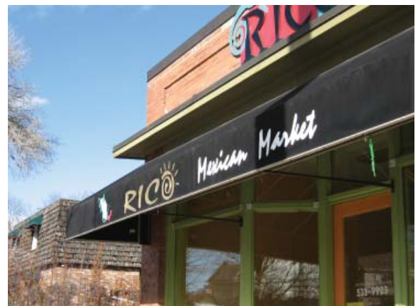
Awnings are generally simple in design, angled and fit within the building opening.
