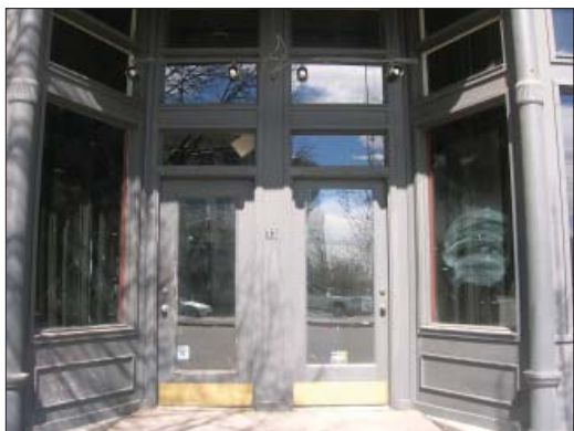
Traditional storefronts consisted of recessed single or double doors flanked by display windows.
