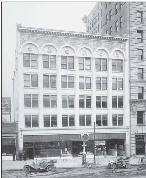
The Felt Building (1910) at 339 S. Main Street displays early use of terra-cotta as a decorative element.
